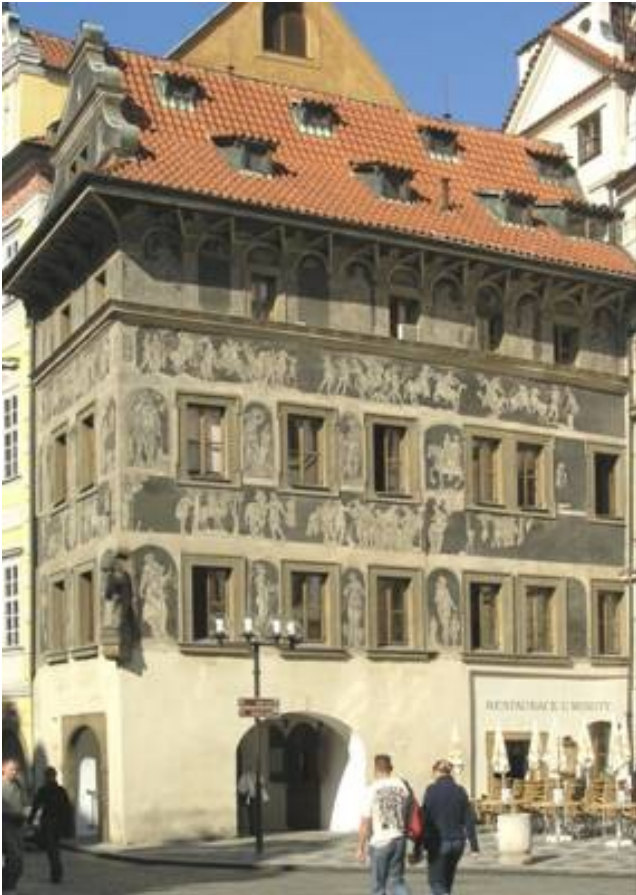
The house at the Old Town Square in Prague
