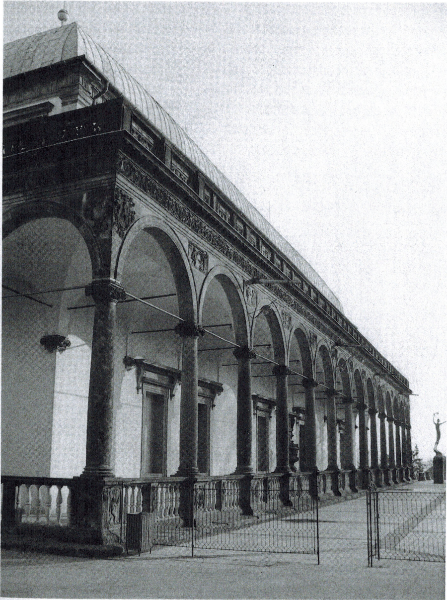
The Royal Summer Palace, Prague Castle, 1537–63, was built by the Italian Paolo della Stella for Ferdinand I, the first Habsburg on the throne of the Bohemian kings. After Paolo's death in 1552, a local architect, Bonifác Wolmut, added the second story and high roof with a conspicuously northern Renaissance double curvature. The building is one of the first echoes of the Italian Renaissance north of the Alps, and its architectural conception and rich sculptural decoration were meant to represent the political ambitions of Ferdinand, who became Holy Roman emperor in 1558. It is one of the earliest examples of the revival of the suburban villa of ancient Rome. The decorative stone reliefs use ancient Roman imagery inspired above all by Virgil's Aeneid to celebrate Ferdinand as the second Jupiter and predestined ruler of the world. Used by permission of Jan Bažant.
