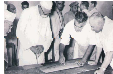
June 6, 1955: Madhya Pradesh Chief Minister Pt Ravi Shankar Shukla pouring over project drawings of Bhilai Steel Plant with Mr SN Mehta General Manager, and Mr Lobotsky, Deputy Chief Engineer
