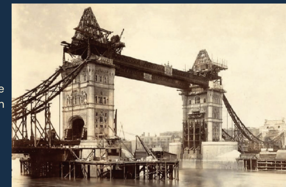
Tower Bridge Construction
