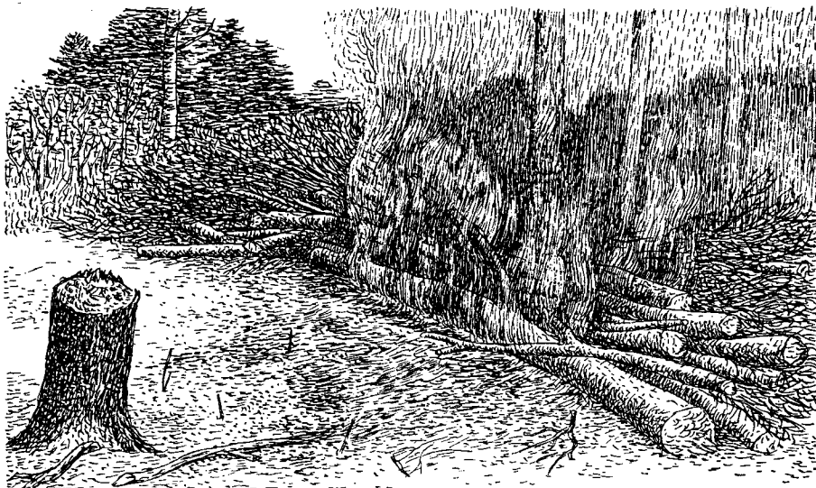
TREES WERE BURNED by covering them with brushwood and igniting a 30-foot strip. When the strip was almost burned out, the larger logs were used to light the next one.
