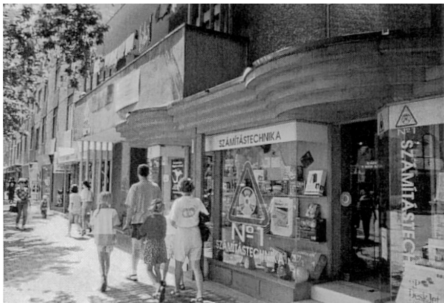
Post-modern facade in ground floor of panel construction housing estate
