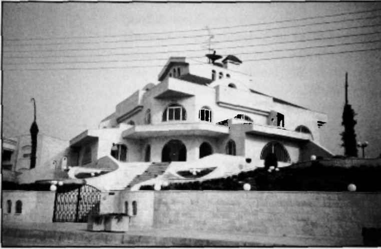
Figure 3. Cottage-style villa, West Amman.
