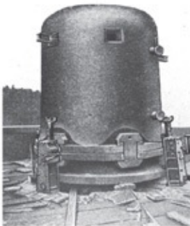
Cloche for Light Machine Gun before installation
