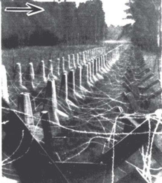
Barrier of Concrete & Iron Hedgehogs - Older Layout
