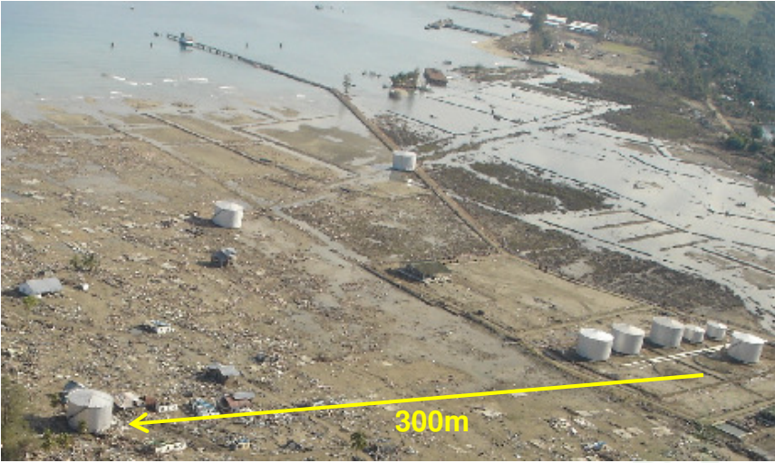
Fig. 1.13 Oil tank carried by the tsunami.
