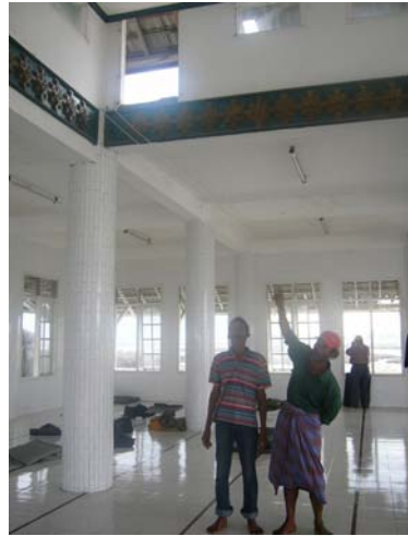
(c) Hole used to escape onto the roof
