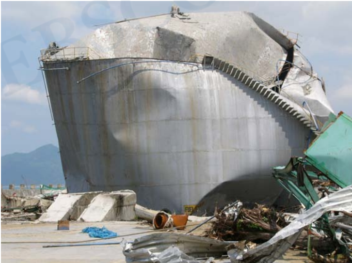
Fig. 1.14 Oil tank heavily deformed by the tsunami.
