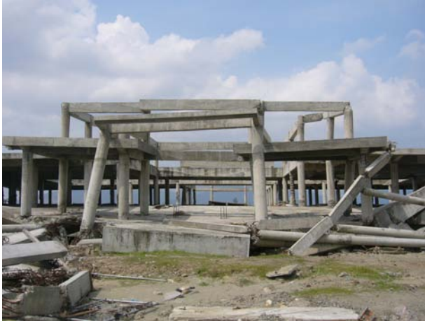
Fig. 1.11 Ferry terminal building under construction, which survived the tsunami.
