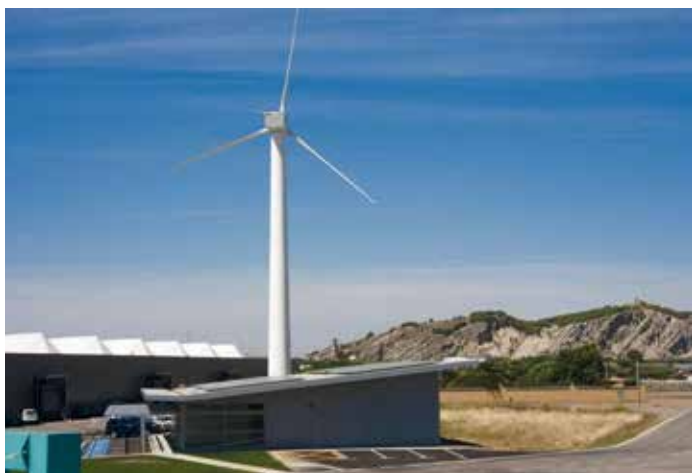
Figure 31 - Factory Microgrid at Jofemar's factory in Peralta (Navarra, Spain)
