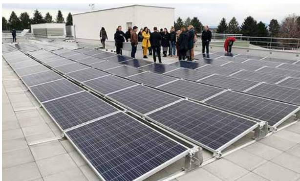
Figure 54 - Križevci Solar Roof: P2P crowdfunding investment model to finance an installation of a 50kW PV system on the rooftop of a business centre owned by the city Križevci (HR)
