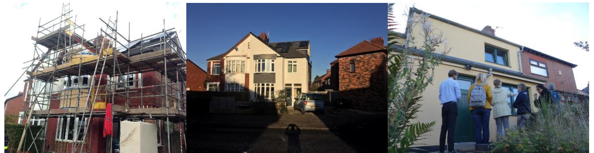
Retrofitting homes in the Greater Manchester Area (©Carbon Co-op)
