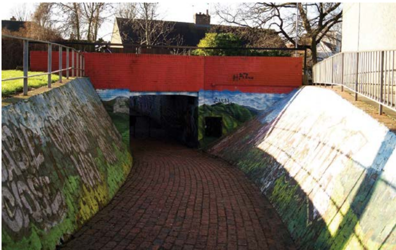
Fig. 3.6 The Beavers Estate tunnel. Source: author
