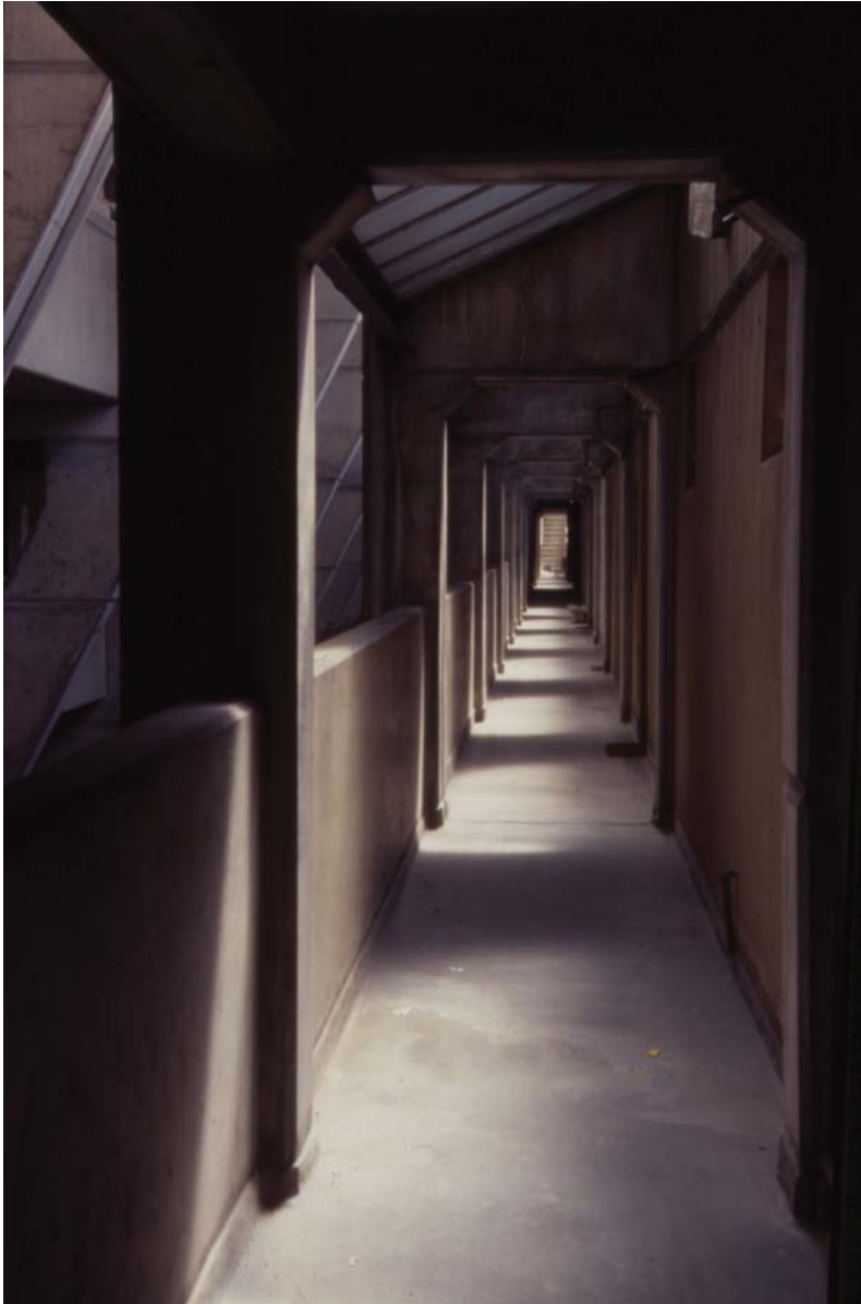
Fig. 2.9 View through second floor access gallery to flats (perimeter block, Foundling Court) 2001. Source: author
