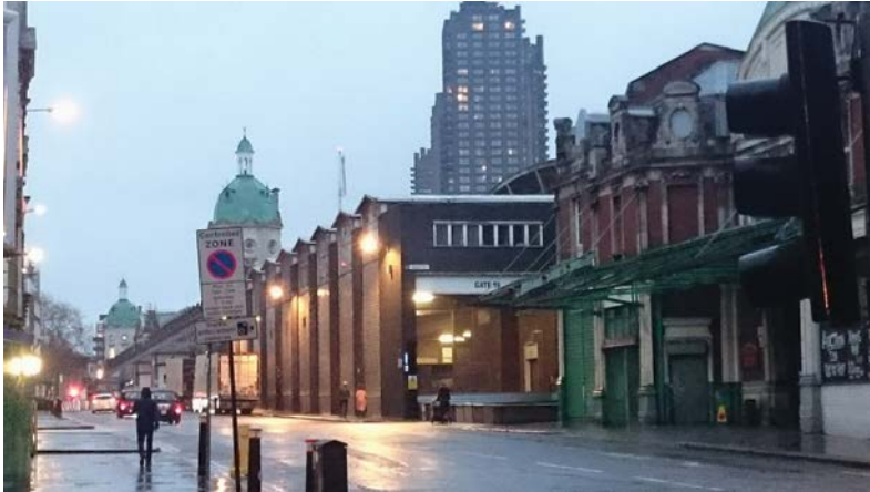
Fig. 6.2 The entire market as seen from west Charterhouse Street. General Market (GM) is in the foreground, followed by Poultry Market (PM), then Main Market (MM) in the background. Source: author
