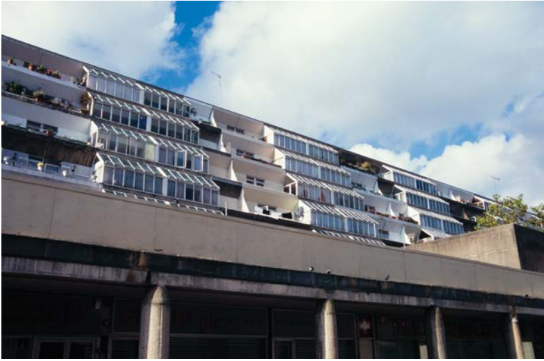
Fig. 2.2 View of winter gardens, O'Donnell Court, prior to 2006 refurbishment. Source: author
