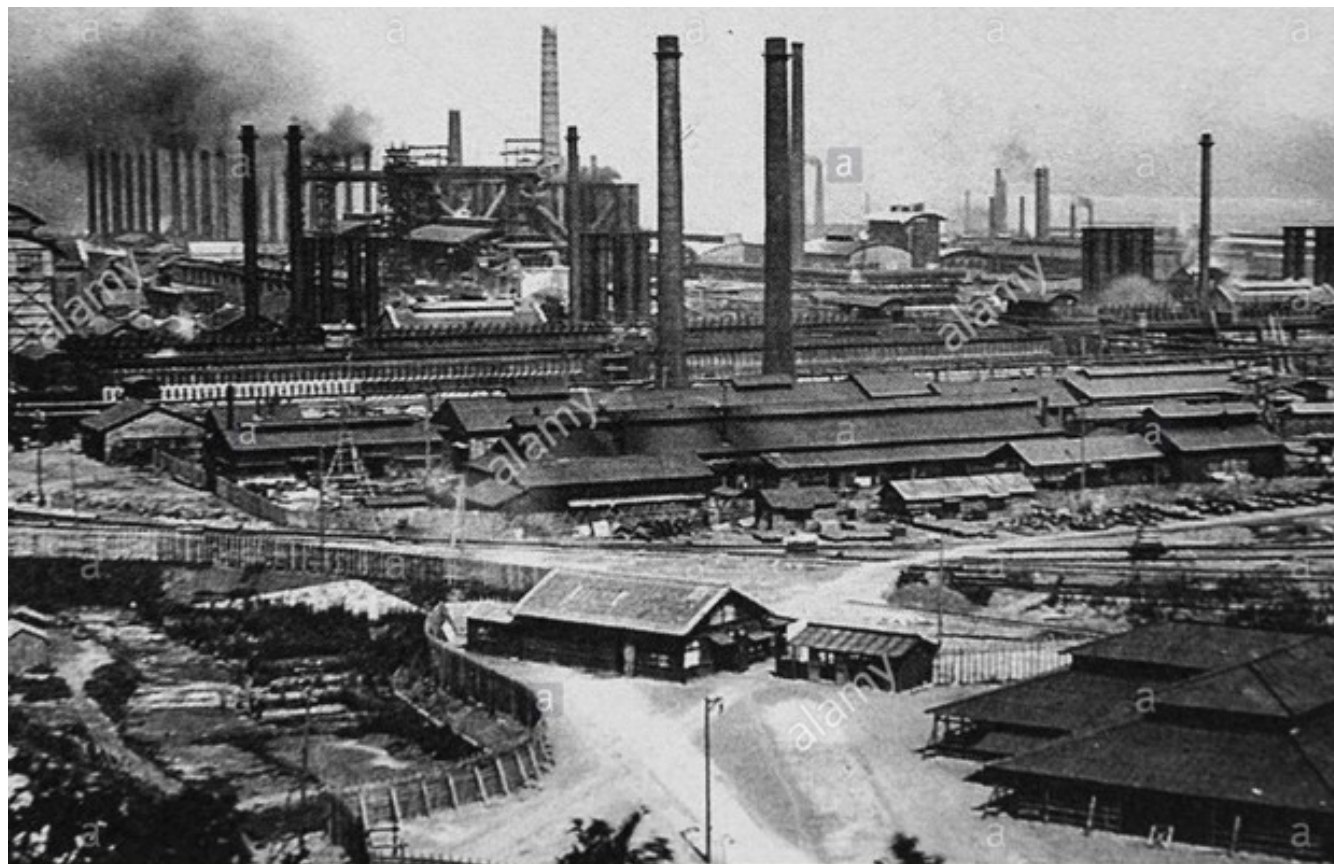
The state-owned Yahata Steel Mill (Kita Kyushu City) was completed in 1901 using German technology with Japanese adjustments
