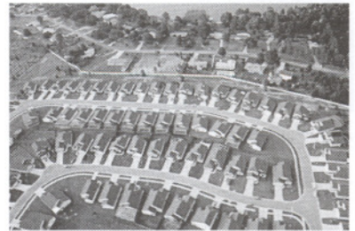
A residential subdivision: houses and parking
