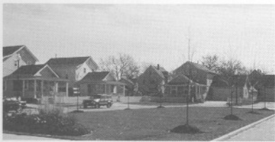
Traditional planning in the traditional city: new low-cost homes (81 in all) blend in with existing houses in central Cleveland
