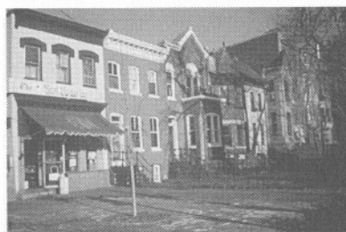
The 7-Eleven as designed by Norman Rockwell: a retail building that is compatible with its residential neighbors
