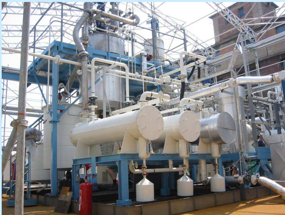
Pilot Plant Erection, Spolana
