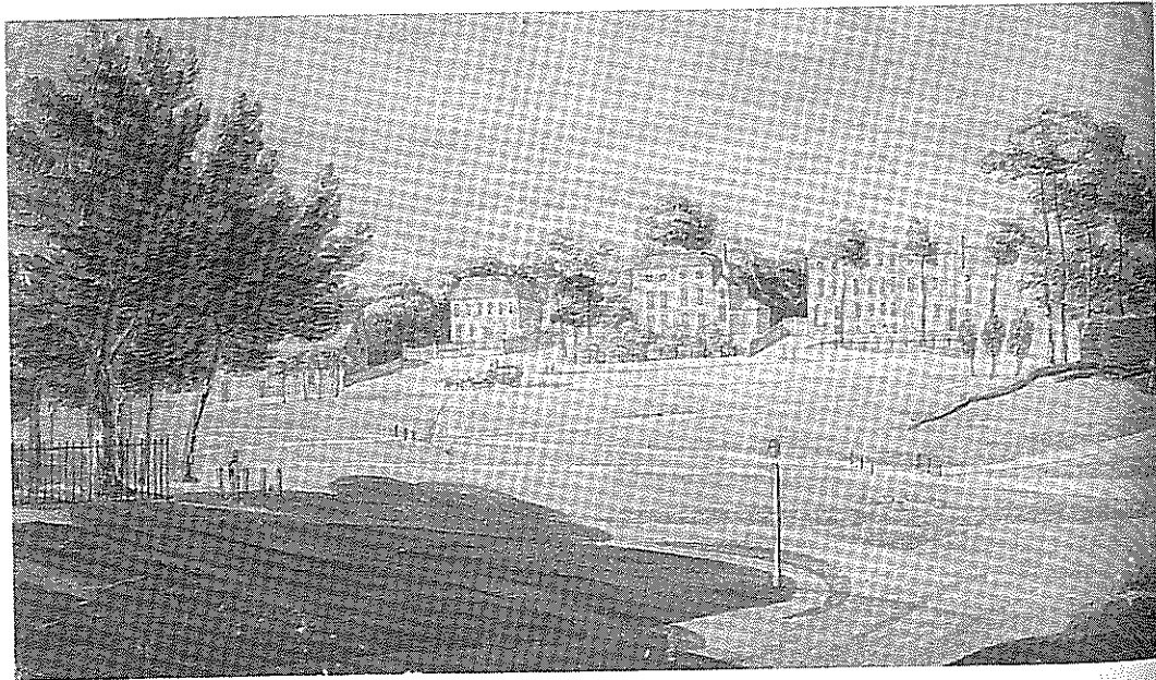
Figure 1-8 This anonymous watercolor in the Guildhall Library depicts Clapham Common circa 1800 with its suburban landscape of large detached villas on lawns sloping down to the Common. Courtesy of Guildhall Library, Corporation of London. Illustration in original.
