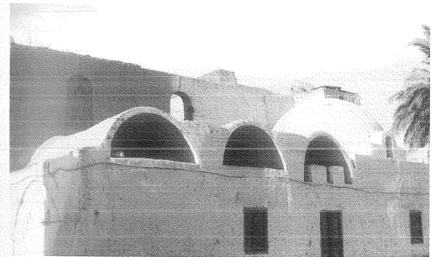
Figure 8.1. The Model Village of New Gurna, built in the 1950s, as photographed in 1999. (Photo by author)
