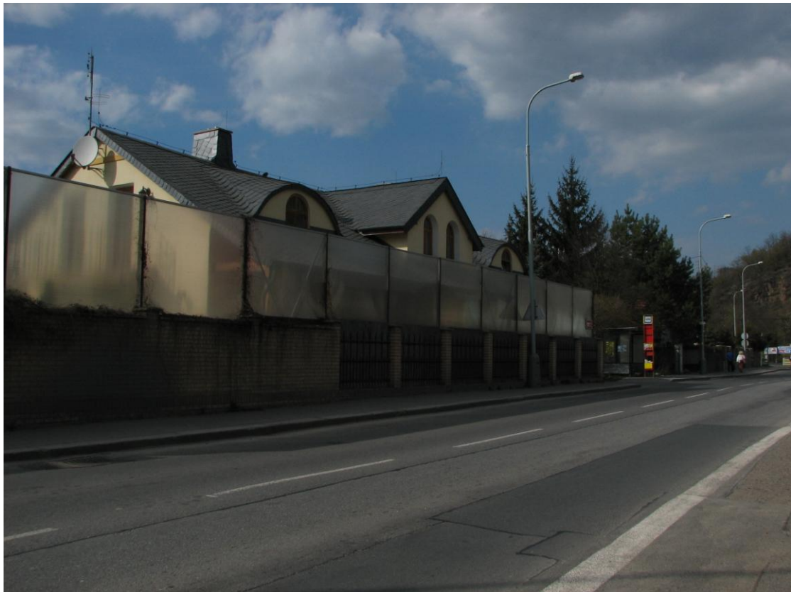
Ill. 5 – The house with an anti-noise barrier
