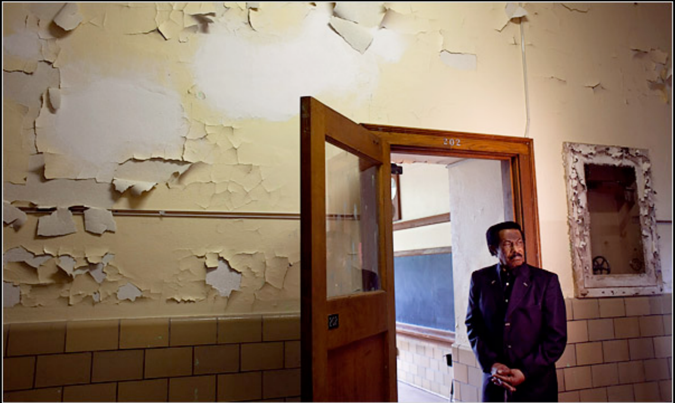
physical space of the classroom
