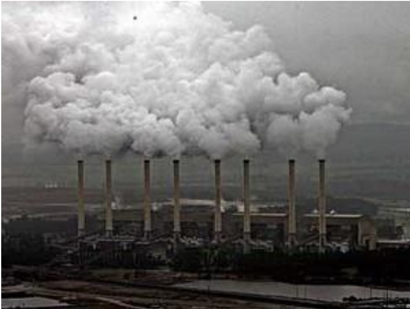
Hazelwood power Station
