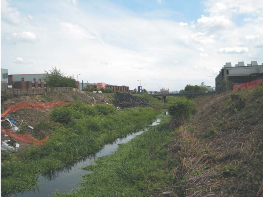
Fig. 3. The Pudding Mill River, tributary of the River Lea, bisecting the southern part of the future Olympic Park. After clearance, the 80,000-seater Olympic Stadium will be located to the left and the warm-up athletics tracks to the right (May 2007) (Source: Authors' photograph).
