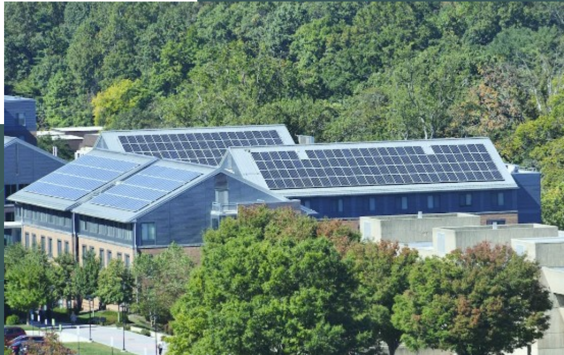
Solar panels on the rooftops of Barton and Douglass Houses.
