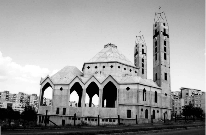
First Cathedral in Dunaújváros, under construction in 1996. Photo: K. Fehérváry.
