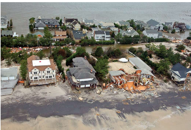
FIGURE 2.7 Coastal damage caused by Hurricane Sandy in Mantoloking, New Jersey. (Courtesy of U.S. Air Force by Master Sgt. Mark C. Olsen— http://www.defense.gov/photoessays/PhotoEssaySS.aspx?ID=3316 , http://www.defense.gov/dodcmsshare/photoessay/2012-10/hires_121030-F-AL508-081c.jpg , Public Domain, https://commons.wikimedia.org/w/index.php?curid=22549477 .)
