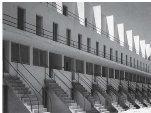
Fig. 18: Alvaro Siza: Bouça publicly assisted housing project, Porto (P), 1977
