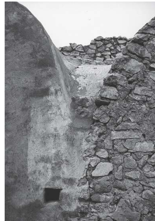
Fig. 64: Ghorfa Detail of partially rendered facade
