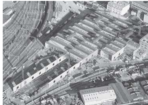
Fig. 65: Aerial view of site, the longest locomotive shed is not yet finished. Herzog & de Meuron: locomotive depot “Auf dem Wolf”, Basel (CH), 1993
