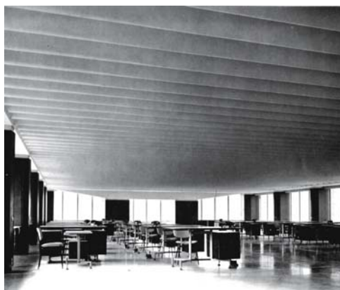
Fig. 9: Galbani office building Milan (I), 1955/56 Reinforced concrete floor by Pier Luigi Nervi Design: E. Soncini, A. Pestalozzo
