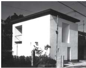
Fig. 95: Hermetically sealed object with shafts apparently driven into the mass Jun Tamaki: Hakama House, Kyoto (J), 1998
