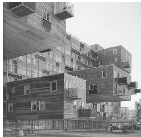
Fig. 66: Steel frame concealed behind timber cladding MVRDV: senior citizens’ apartments, Amsterdam (NL), 1997
