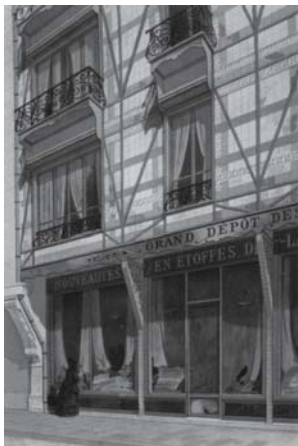
Fig. 4: View of building with iron frame Viollet-le-Duc: coloured plate from Entretiens sur l'architecture , 1812
