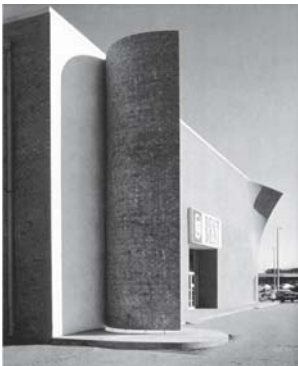
Fig. 12: Brick wall as peel-off skin! SITE: Peeling Project (Best department store), Richmond, Virginia (USA), 1971–72
