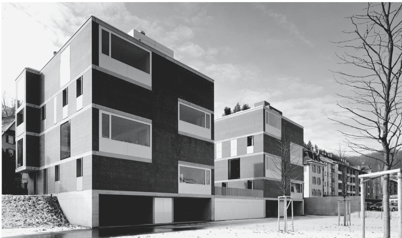
Fig. 35: View from the "Merker" meadow The difference in levels reveals the basement.
