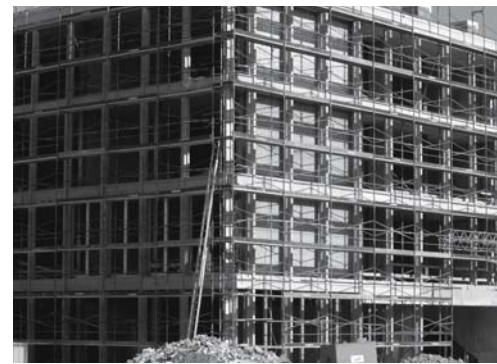
Fig. 224: View during construction
