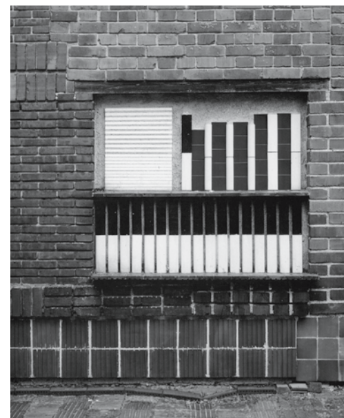
Figure 61: Various formats, colours and surface textures Alvar Aalto: experimental house, Muuratsalo (FIN), 1954
