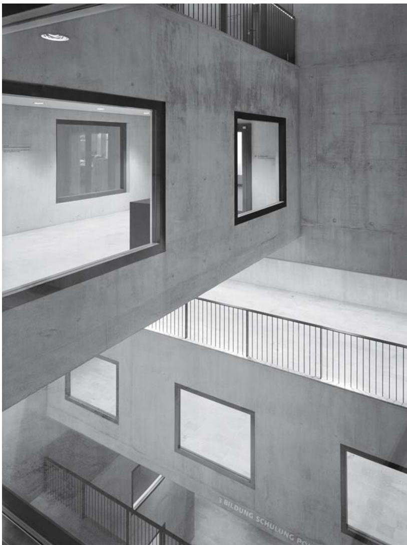
Fig. 192: Upper atrium, looking down towards entrance level The walls without intermediate supports act as storey-high deep beams.
