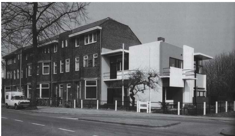
Fig. 10: Roadside elevation showing the entrance at the side Gerrit Rietveld: Rietveld-Schröder House, Prins Hendrikklaan 50, Utrecht (NL), 1924
