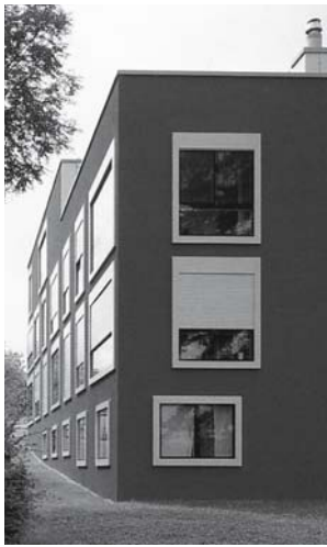
Fig. 77: The components of the sunshading system are housed behind an aluminium fascia and are therefore concealed when not in use. Gigon/Guyer: Bröelberg development, Kilchberg (CH), 1996
