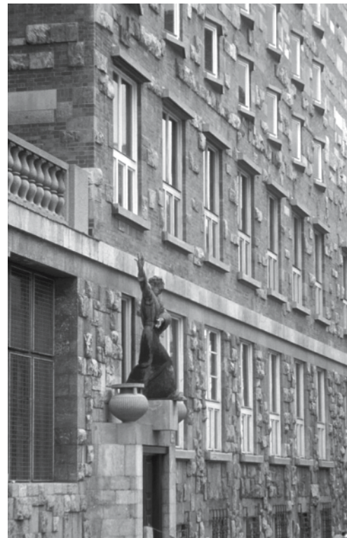
Fig. 5: A weave of natural stone and clay bricks Jože Plečnik: University Library, Ljubljana (SLO), 1941
