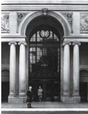
Fig. 52: The revolving door as a trademark of a grand hotel, Olive Street entrance, The Biltmore Hotel, Los Angeles (USA), 1923
