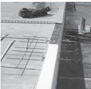
Fig. 33: Example of insulated reinforcement being installed
