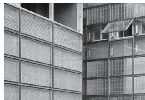
Fig. 2: Existing and new buildings linked by insulating glass facade; top: straight on the road side; bottom: diagonally in the inner courtyard Herzog & de Meuron: Suva combined residential and commercial development, Basel (CH), 1988–93
