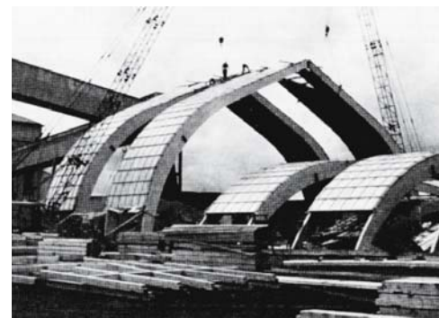
Fig. 121: Erection of prefabricated half-shells Salt warehouse
