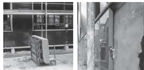
Fig. 49: Stone facade Fixed with cast-in dowels
