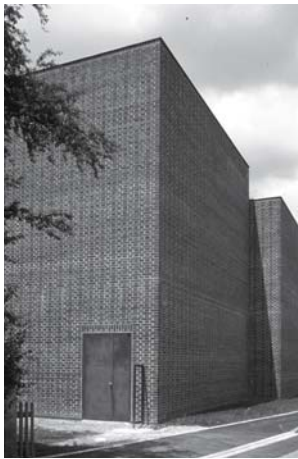
Figure 68: Solid masonry without additional layer of insulation Bearth & Deplazes: Gallery for Contemporary Art, Marktoberdorf (D), 2001
