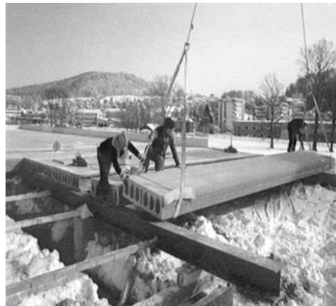
Fig. 6: The concrete elements are lifted into position with a crane.
