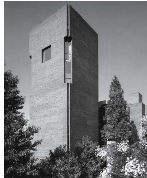
Fig. 44: Wall panels joined by diagonal corner window "hinge" Louis Kahn: Richards Medical Research Centre, Philadelphia (USA), 1965
