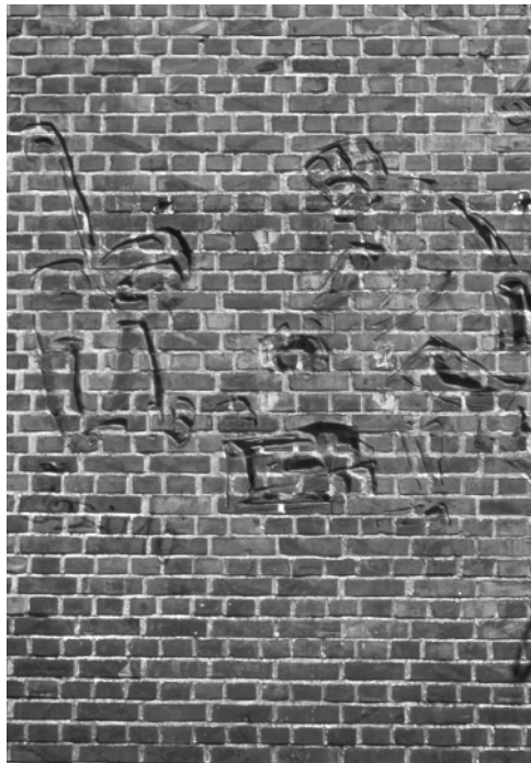
Fig. 19: Decoration cut into brickwork after erection Theodor Fischer: Ledigenheim, Munich (D), 1927
