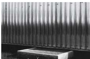
Fig. 62: The lightwell as an indication of a basement Marques & Zurkirchen: Kraan-Lang House, Emmenbrücke (CH), 1994
