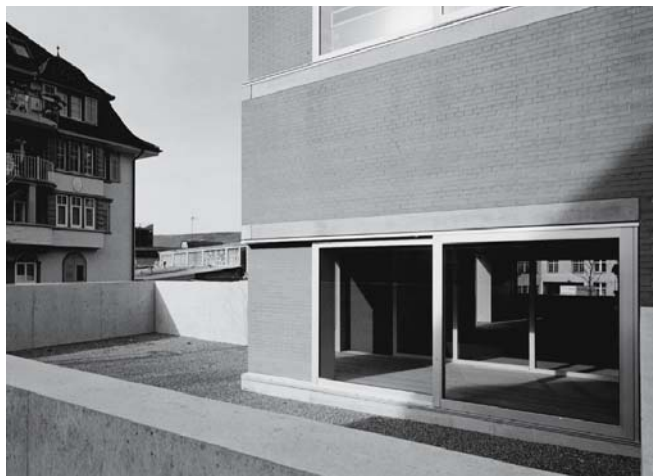
Fig. 61: Ground floor veranda The sliding doors opening onto the veranda lend depth to the facade.
