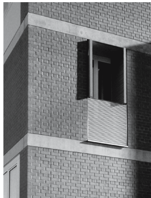
Fig. 55: Close-up of French window Weatherproof screen acts as balustrade and shutter.
