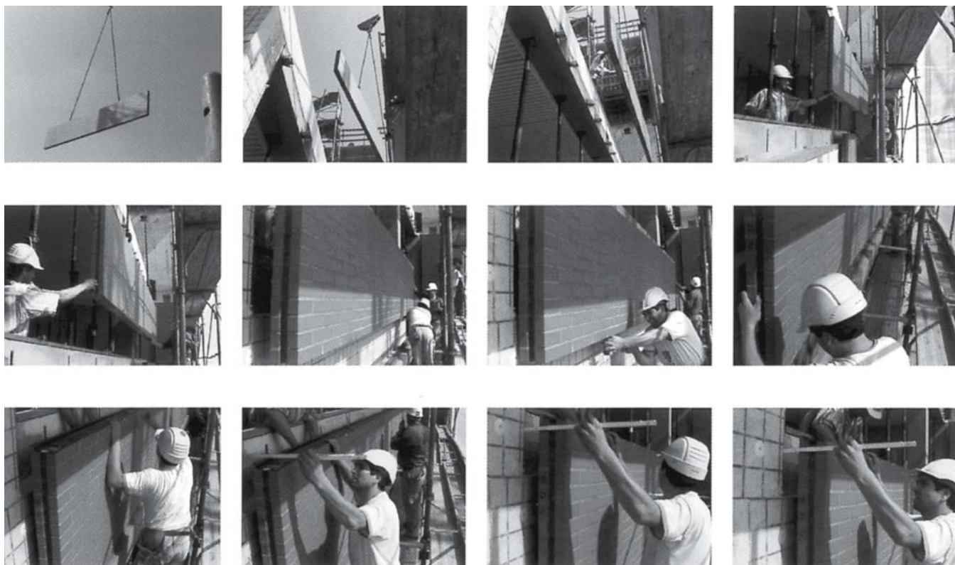
Fig. 77: Examples from a Swiss manufacturer: "preton" element catalogue Masonry elements being erected at the Swisscom headquarters by Burkard, Meyer in Winterthur
