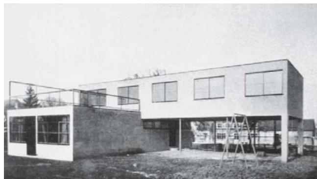
Fig. 114: All traces of the structure are concealed behind masonry panels and render. Artaria & Schmidt: Schaeffer House, Riehen (CH), 1927–28
