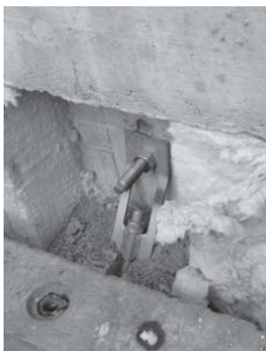
Fig. 43: Heavy external cladding
