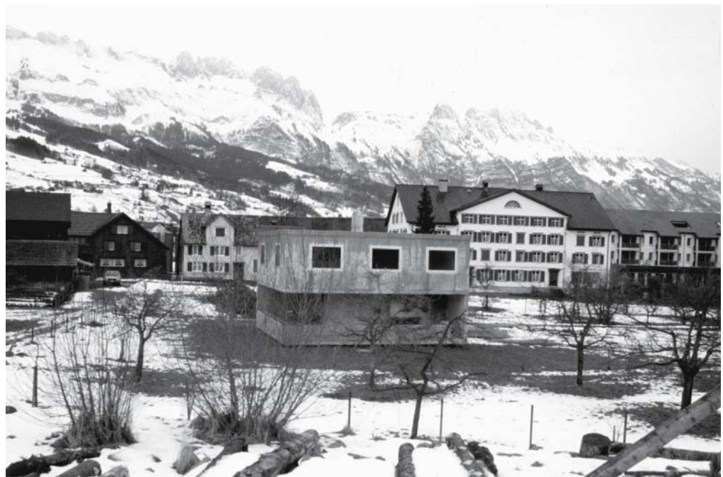
Fig. 93: The house stands like sculpture on the open ground.
