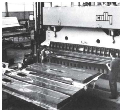
Fig. 15: Industrial manufacture of facade elements: individual parts of element Jean Prouvé: CIMT, Paris (F), c. 1955
