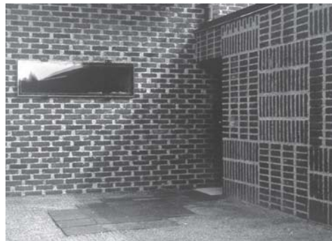
Figure 65: Joint and bond used to create an autonomous image Sigurd Lewerentz: St Peter's Church, Klippan (S), 1966
