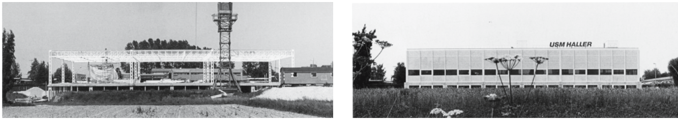
Fig. 118: MAXI steel building system, (above) before adding the cladding, (right) with associated facade system Fritz Haller: USM plant, Bühl (D), 1983–87
