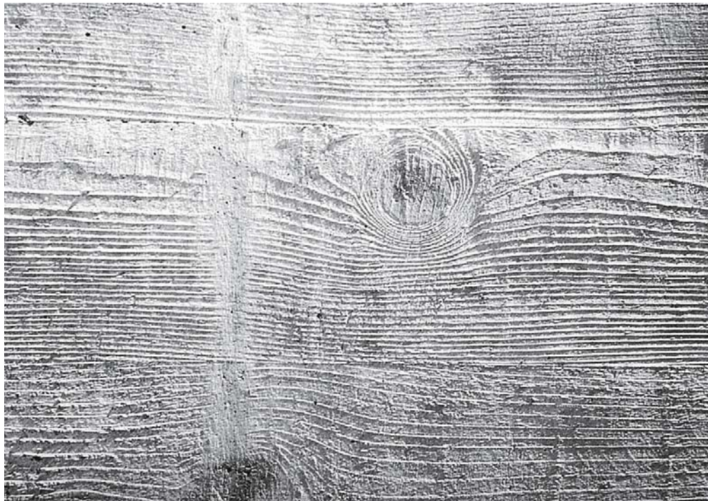
Fig. 1: Formwork “fingerprint” Rough-sawn boards
