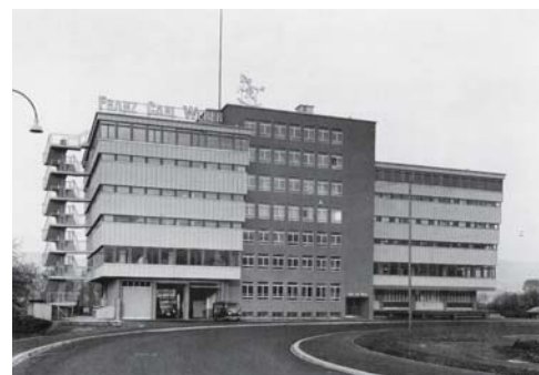
Fig. 124: Facade using Durisol system Rudolf Kuhn and Heinz Ronner: FCW warehouse, Zurich (CH), 1954–55
