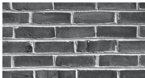
Fig. 26: The presence of the material is strengthened by using distorted, "reject" bricks. Alvar Aalto: Baker House, Massachusetts Institute of Technology, Cambridge (USA), 1954
