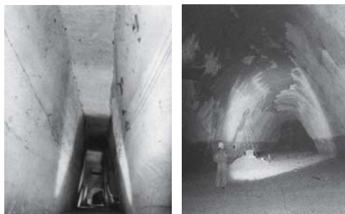
Fig. 20: Vaults in tuff stone, Naples Trapezoidal (left) and elliptical (right) cross-sections as structurally ideal forms
