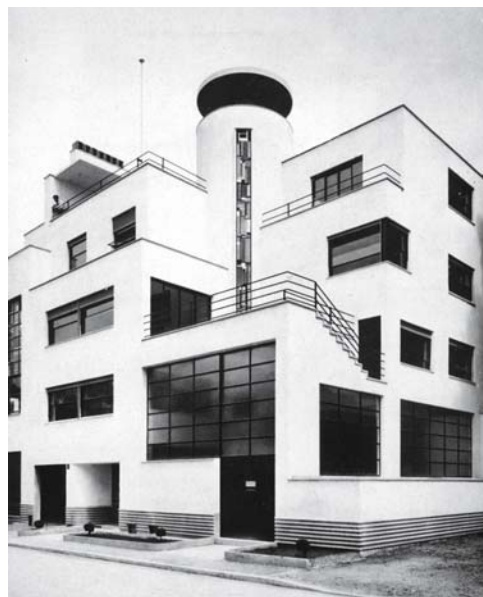
Fig. 105: External view with studio in foreground and exposed staircase core
