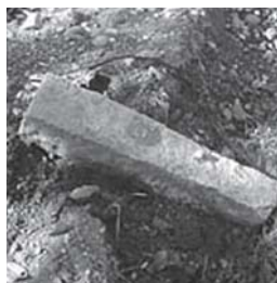
Fig. 37: Boundary stone prior to installation
