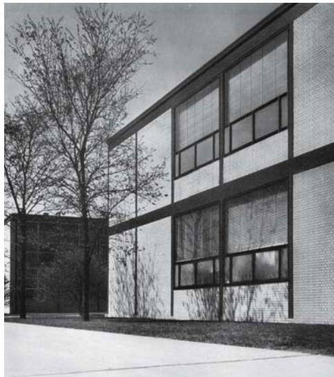
Fig. 13: The exposed steel columns support the masonry only. Ludwig Mies van der Rohe: Illinois Institute of Technology, Chicago (USA), 1940–50
