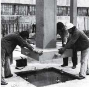
Fig. 33: Erecting a steel column
