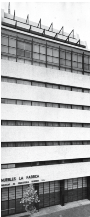
Fig. 36: Different horizontal strip windows lend the facade a distinct hierarchy. M. Ponsett, E. Salas: "La Fabrica" furniture manufacturer, Barcelona (E), 1961
