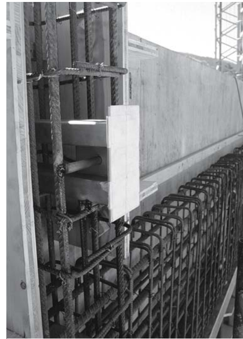
Fig. 136: Cage of reinforcement with shear stud positioned ready for cast-
