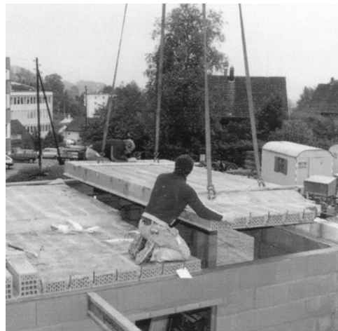
Fig. 1: Top: hollow clay blocks and reinforced concrete ribs; bottom: erection of factory-prefabricated elements (here: Bricosol products)
