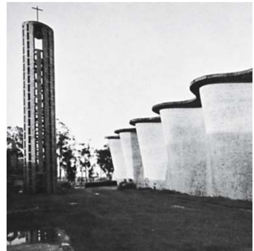
Fig. 24: Curving brickwork shells Eladio Dieste: Church in Atlántida (Uruguay), 1960
