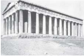
Fig. 55: The plinth as a platform to prepare the site Greek temple, c. 500 BC
