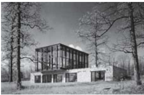
Fig. 57: Substructure and superstructure as structurally independent constructions with the same use (residential) Philip Johnson: Wiley House, New Canaan (USA), 1953
