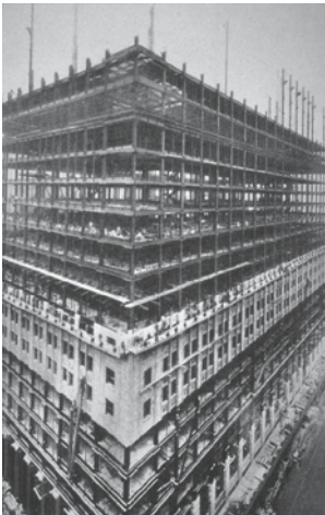
Fig. 6: Chicago The steel frame to a „solid“ high-rise block
