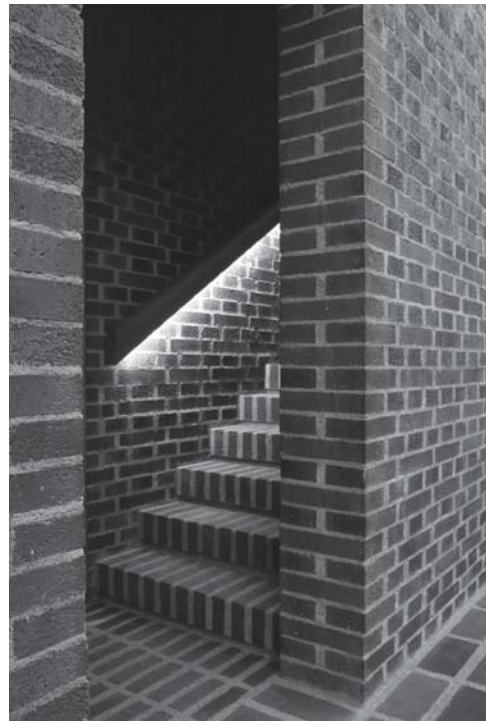
Fig. 72: Masonry enclosing walls
