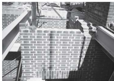
Fig. 75: Bearing for floor beam
