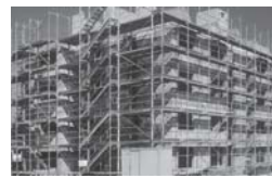
Fig. 5: Structural shell Masonry building, under construction
