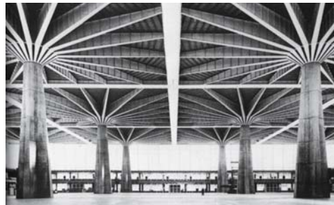
Fig. 76b: Canopies of concrete and steel, bay size 38 x 38 m Pier Luigi Nervi: Hall of Labour, Turin (I), 1961
