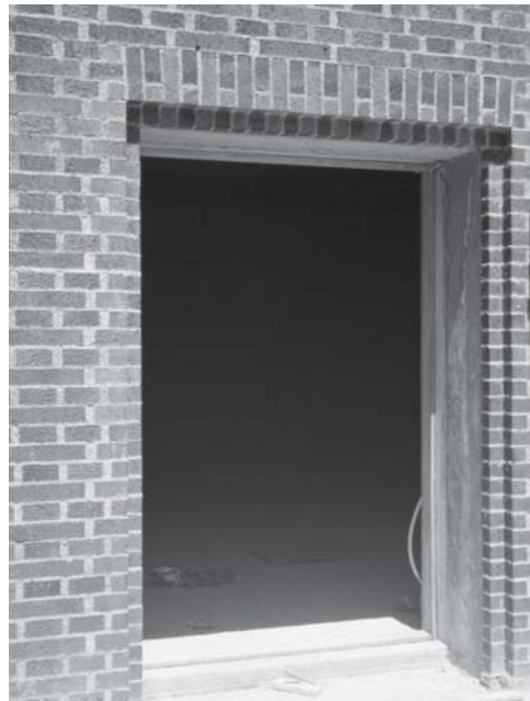
Fig. 77: Special reveal bricks prior to fitting door
