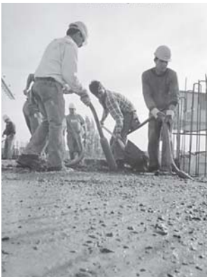
Fig. 18: Compacting the concrete
