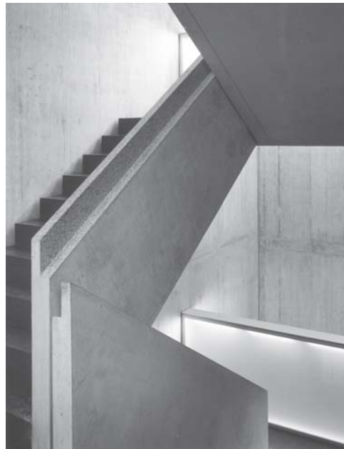
Fig. 32: Staircase Burkhard Meyer & Partner: Service centre, Winterthur (CH), 1999
