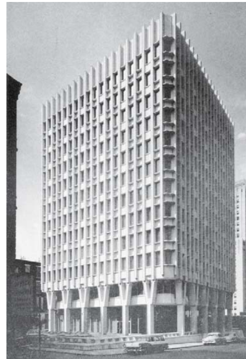
Fig. 23: Amalgamation of loadbearing structure and vertical service ducts Paul Rudolph, with Anderson, Beckwith & Haible: Blue Cross Building, Boston (Mass., USA), 1958
