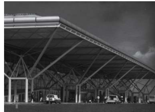
Fig. 79: Modular roof; a second element is suspended between the columns. Norman Foster: Stansted airport, London (GB), 1991
