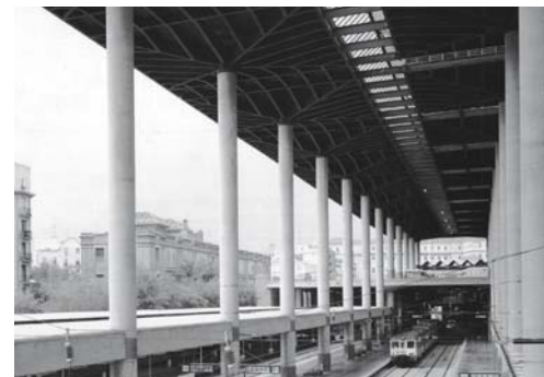
Fig. 80: The structure is legible both internally and externally. Rafael Moneo: Atocha station, Madrid (E), 1984–92
