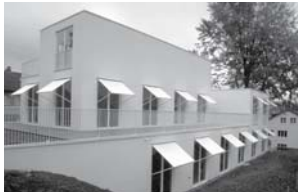
Fig. 9: Oliver Schwarz architectural practice: Peter apartment block, Rüslikon (CH), 1997
