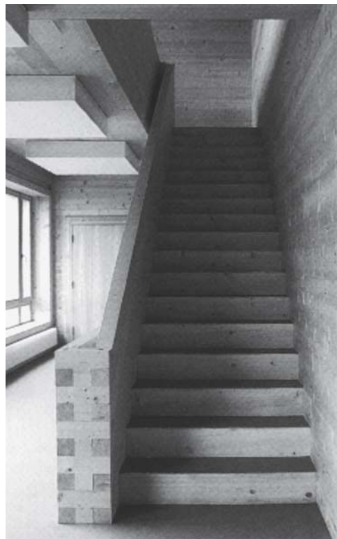
Fig. 46: General view of stair
