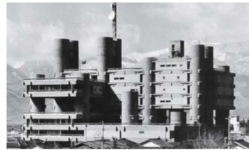
Fig. 5: Loadbearing structure and infrastructure combined in shafts Kenzo Tange: communications centre, Kofu (J), 1964–67
