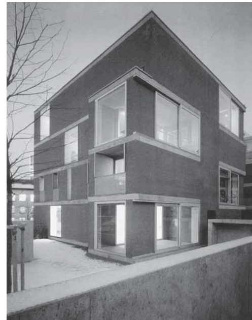
Fig. 45: External view of block A The garden wall along Martinsbergstrasse can be seen in the foreground.
