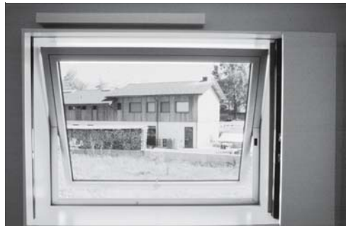
Fig. 122: Horizontal pivot window from inside
