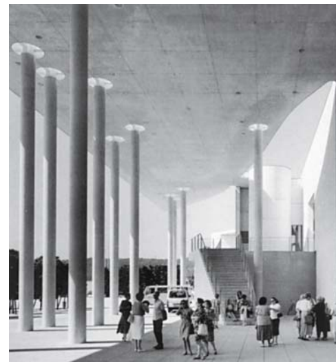
Abb. 54: Spun-concrete columns, connected to reinforced concrete roof via steel web plates. Axel Schultes: art gallery, Bonn (D), 1992
