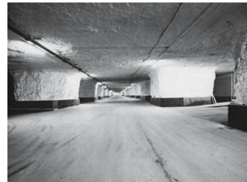
Fig. 26: Solid rock hollowed out to create a cold store and warehouse Great Midwest Underground, started in and continually expanded since 1940, Kansas City (Missouri, USA)
