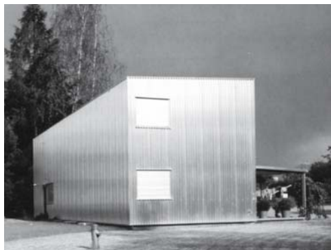
Fig. 63: A container without an anchorage, “temporarily” parked on the grass Marques & Zurkirchen: Kraan-Lang House, Emmenbrücke (CH), 1994
