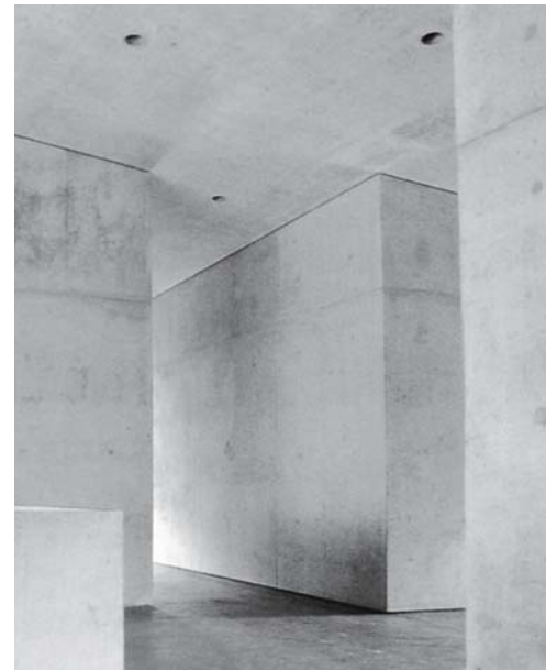
Fig. 141: Corridor, 2nd floor
