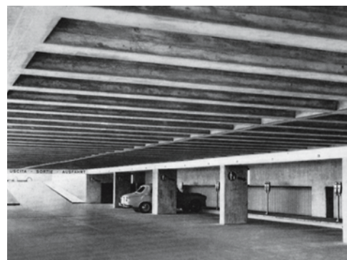
Fig. 62: Basement garage, c. 1960 Ribbed slab
