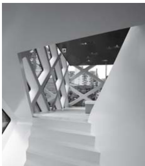
Fig. 73: Rhombus-shaped loadbearing structure to facade Herzog & de Meuron: Prada store, Tokyo (J), 2003
