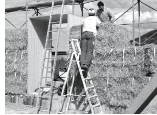
2 Building up the wall with straw bales in a "masonry bond"
