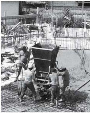
Fig. 21: Placing concrete by crane skip
