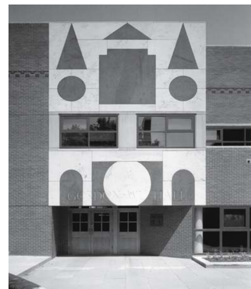
Fig. 13: Entrance beneath fascia of marble and grey granite. The motifs are reminiscent of the early Renaissance and emphasise the central transition to the building.
