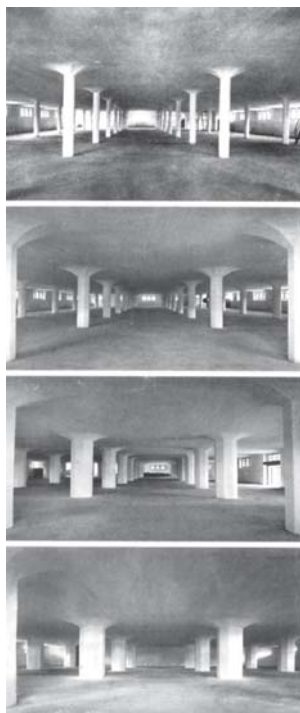
Fig. 1: Flared-head columns in reinforced concrete (diameter varies with storey, or rather load) Robert Maillart: grain warehouse, Altdorf (CH), 1912
