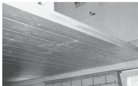
Fig. 8: Staggered positioning of solid timber elements
