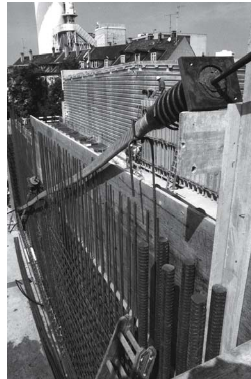
Fig. 162: Shear wall showing reinforcement and prestressing tendon
