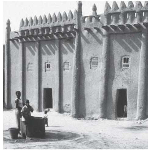
Fig. 30: Cob construction with timber reinforcement (internal frame) with protective covering of cob (transverse ribs) Traditional construction of the Dogon people (Mali)
