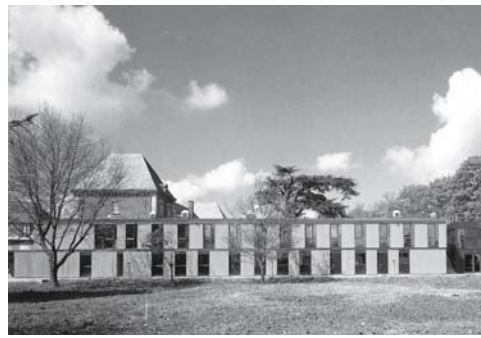
Fig. 127: Storey-high clay elements with loadbearing and insulating functions; (left) erection of loadbearing structure at ground floor level, (above) finished building
