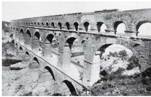
Fig. 36: Succession of stacked arches: sectional concept in order to omit superfluous material. The arch construction is sensible from an engineering and an economic viewpoint.
