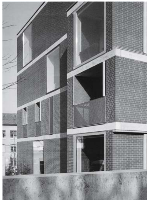
Fig. 4: Flexibility in planning: the position of the windows was determined by the buyers of the apartments. Burkard, Meyer: apartment blocks, Martinsbergstrasse, Baden (CH) 1998/99
