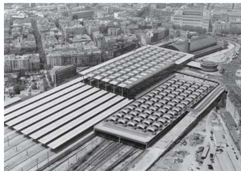
Fig. 78: The table-like construction lends texture to the trainshed roof. Rafael Moneo: Atocha station, Madrid (E), 1984–92
