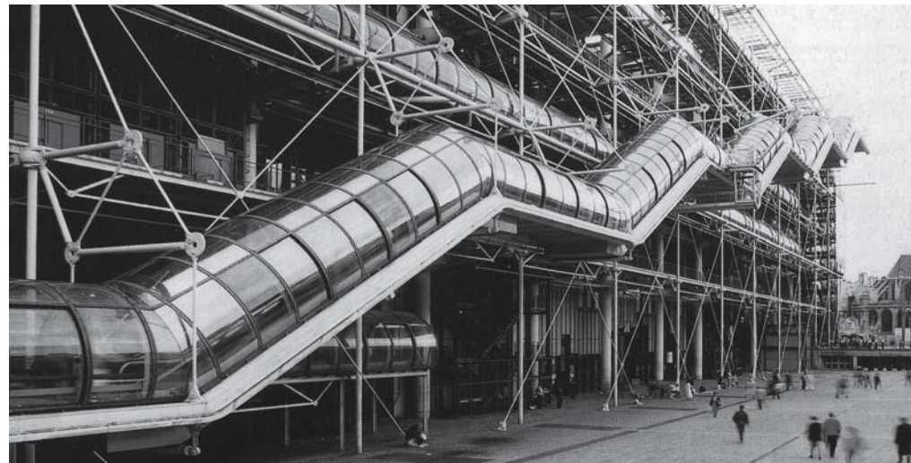
Fig. 22: Exposed infrastructure as the characterising motif Renzo Piano & Richard Rogers: Centre Pompidou, Paris (F), 1971–78
