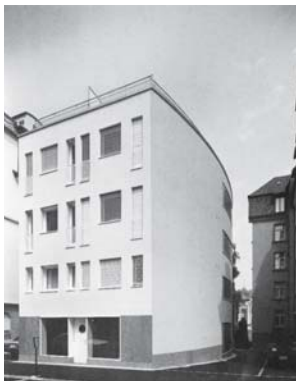
Fig. 66: Rendered thermal insulation with stone plinth Dolf Schnebli: apartment block, Baden (CH), 1990
