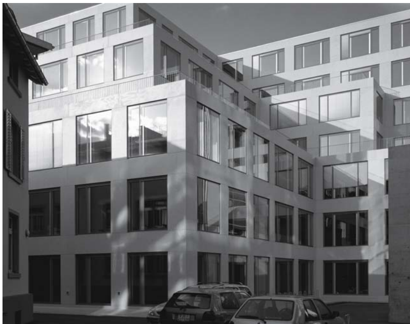
Fig. 178: View of rear of building
