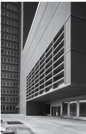
Fig. 13: Prefabricated brickwork panels Urs Burkhard, Adrian Meyer: Swisscom head- quarters, Winterthur (CH), 1999
