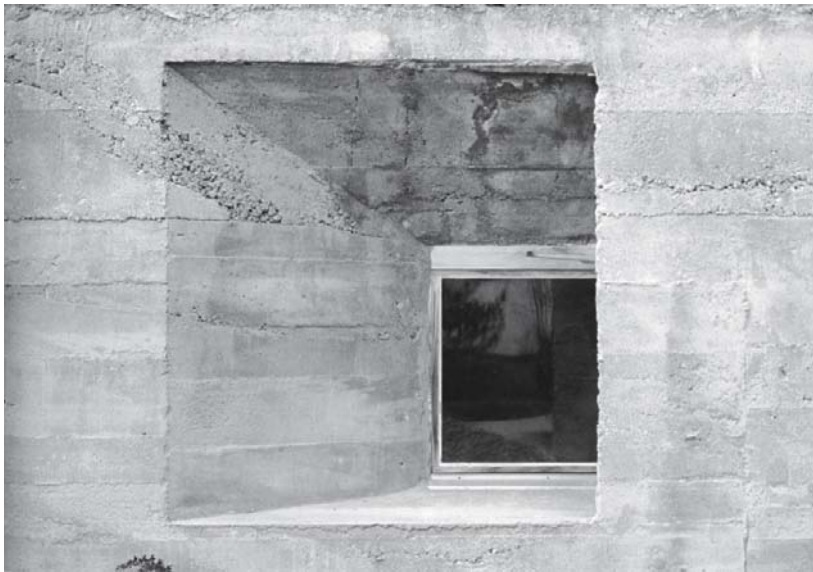
Fig. 22: Timber boards and honeycombing result in rough surfaces Rudolf Olgiati: house for Dr G. Olgiati, Flims-Waldhaus (CH), 1964–65
