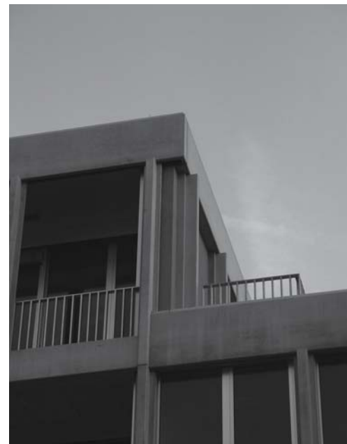
Fig. 220: Corner of building and edge of roof Steel safety barrier to escape balcony, glazing and rendered brick wall
