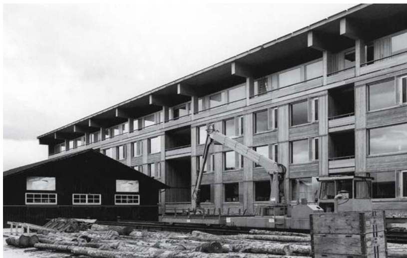
Figs 256 and 257: The Swiss School of Engineering for the Wood Industry is a series of wooden boxes.
