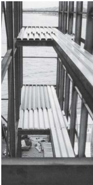
Fig. 37: Composite floor construction Profiled metal sheeting prior to concreting
