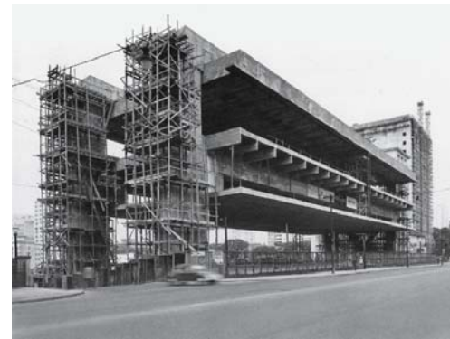
Fig. 33: Frame with suspended floors Lina Bo Bardi: Museum of Modern Art, São Paulo (BR), 1957–68
