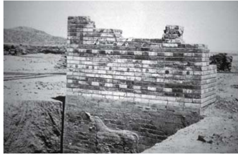
Fig. 2: The wall as a boundary element is the primary function, the masonry as loadbearing element the secondary function. Nineveh, excavations of town walls between 1899 and 1917
