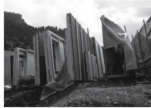
Fig. 297: Timber platform frame elements waiting to be erected The timber platform frame construction was erected in two days.
