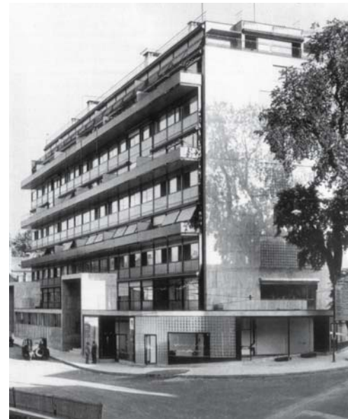
Fig. 12: Windows positioned as panels between steel frame members Le Corbusier & Pierre Jeanneret: Maison Clarté, Geneva (CH), 1932
