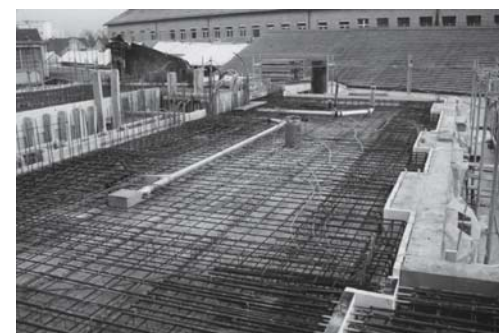
Fig. 52: 1st floor slab The returns in the slab edge elements indicate the positions of the French windows.
