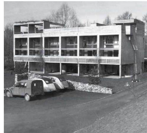
Fig. 109: The south facade reflects the shear wall structure. Atelier 5: Flamatt 1 residential development, Bern (CH), 1957–58
