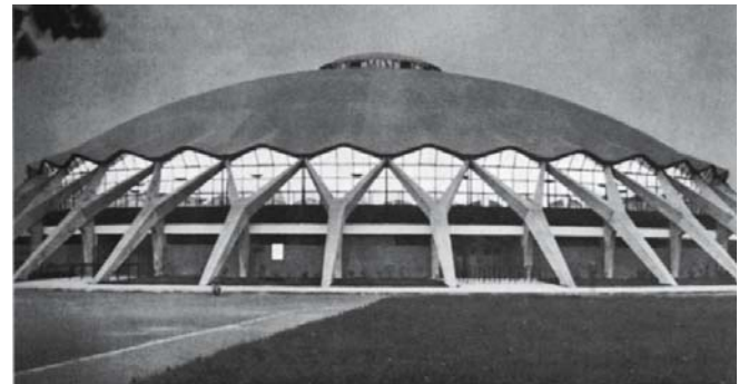
Fig. 44: The dome is resolved into a ring of Y-shaped raking columns Pier Luigi Nervi: Palazzetto dello Sport, Rome (I), 1957
