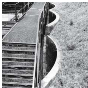
Fig. 28: Retaining wall with “arch” form to resist earth pressure Tank compound, aluminium works, Chippis (CH)
