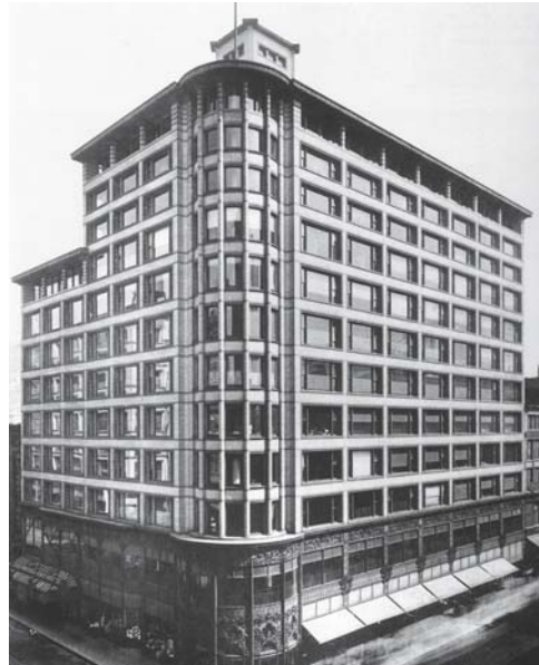
Fig. 6: The opening–wall ratio points to a frame behind the facade. Louis Henry Sullivan: Schlesinger & Mayer department store, Chicago (USA), 1904
