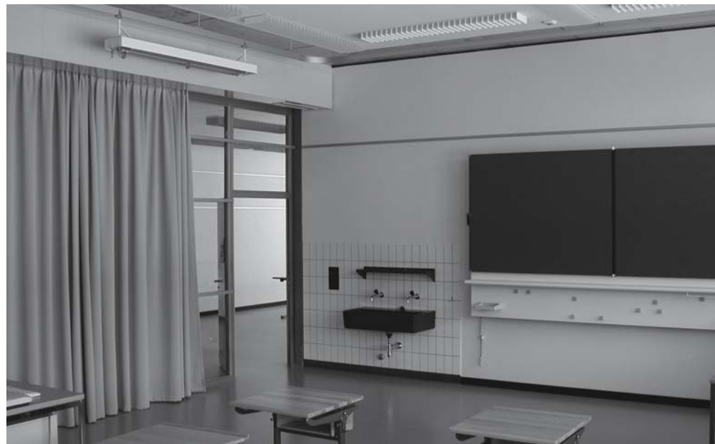
Fig. 234: Materials in classroom Fair-face concrete soffit and acoustic gypsum panels with integral lighting units, ventilation duct clad with grey sheet metal, glazing with curtains, peripheral aluminium rail for displaying drawings etc., sink and blackboard, beige-coloured linoleum floor covering
