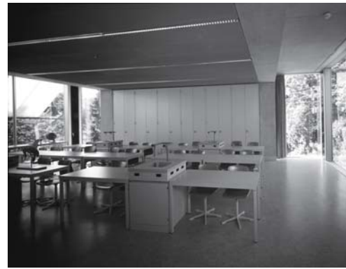
Fig. 240: Seminar room A suspended ceiling between the downstand beams, but only the bare concrete soffit adjacent to the facade (see section)
