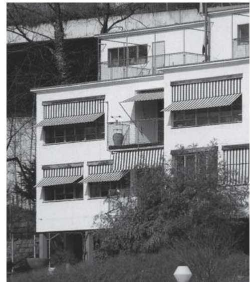
Fig. 83: Semi-awnings to the windows, straight-arm awnings and vertical blinds to the balconies Max Ernst Haefeli: Rotach development, Zurich (CH), 1928
