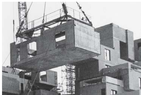
Fig. 135: The units are erected as “structural shells” without any roof. Moshe Safdie: HABITAT 67, Montreal (CAN), 1966–67
