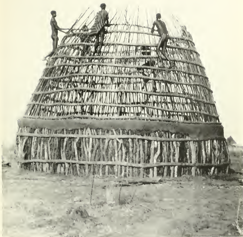
Building a cattle byre (Eastern Jikany)
