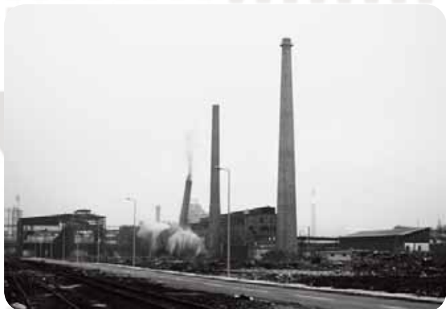
Three out of sixteen chimneys at the largest steel plant in the former Yugoslavia being demolished in March 2008.
