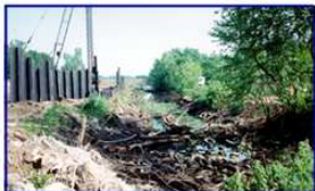
The East Ditch, located at the south, contained discarded tires and debris.
