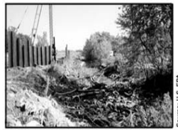
The East Ditch, located at the south end of Bowers Landfill, contained discarded tires and debris.
