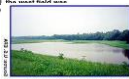
1993: The embankment area with vegetation cover, resulting in erosion and debris removal.
