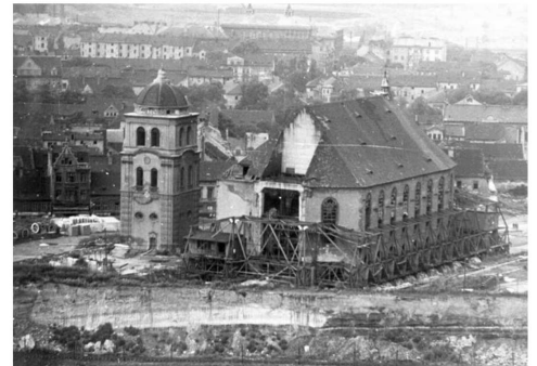
Transport on rails 841m outside the occurrence of coal
