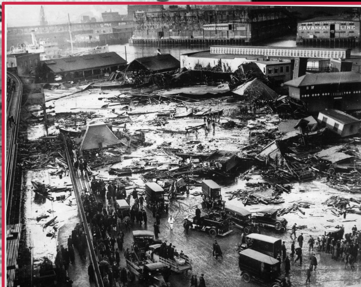
GENERAL VIEW OF THE WRECK OF THE NORTH END TANK, SHOWING SOME OF THE DESTRUCTION AND THE MESS OF THE WRECK. THE TANK WAS BUILT BY THE BOSTON TANK CO. AND WAS USED FOR THE STORAGE OF MOLASSES. THE TANK WAS 100 FEET HIGH AND 100 FEET IN DIAMETER. IT WAS BUILT IN 1908 AND WAS THE LARGEST TANK OF ITS KIND IN THE WORLD. THE TANK WAS BUILT BY THE BOSTON TANK CO. AND WAS USED FOR THE STORAGE OF MOLASSES. THE TANK WAS 100 FEET HIGH AND 100 FEET IN DIAMETER. IT WAS BUILT IN 1908 AND WAS THE LARGEST TANK OF ITS KIND IN THE WORLD.
