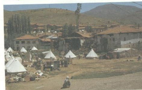
Damaged houses after an earthquake in Turkey
