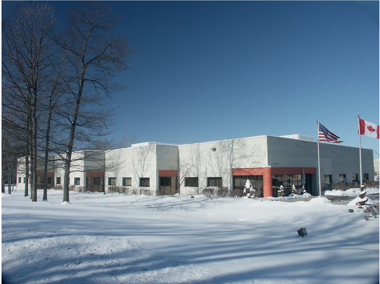
Industrial - Small Factory in Troy, Michigan
