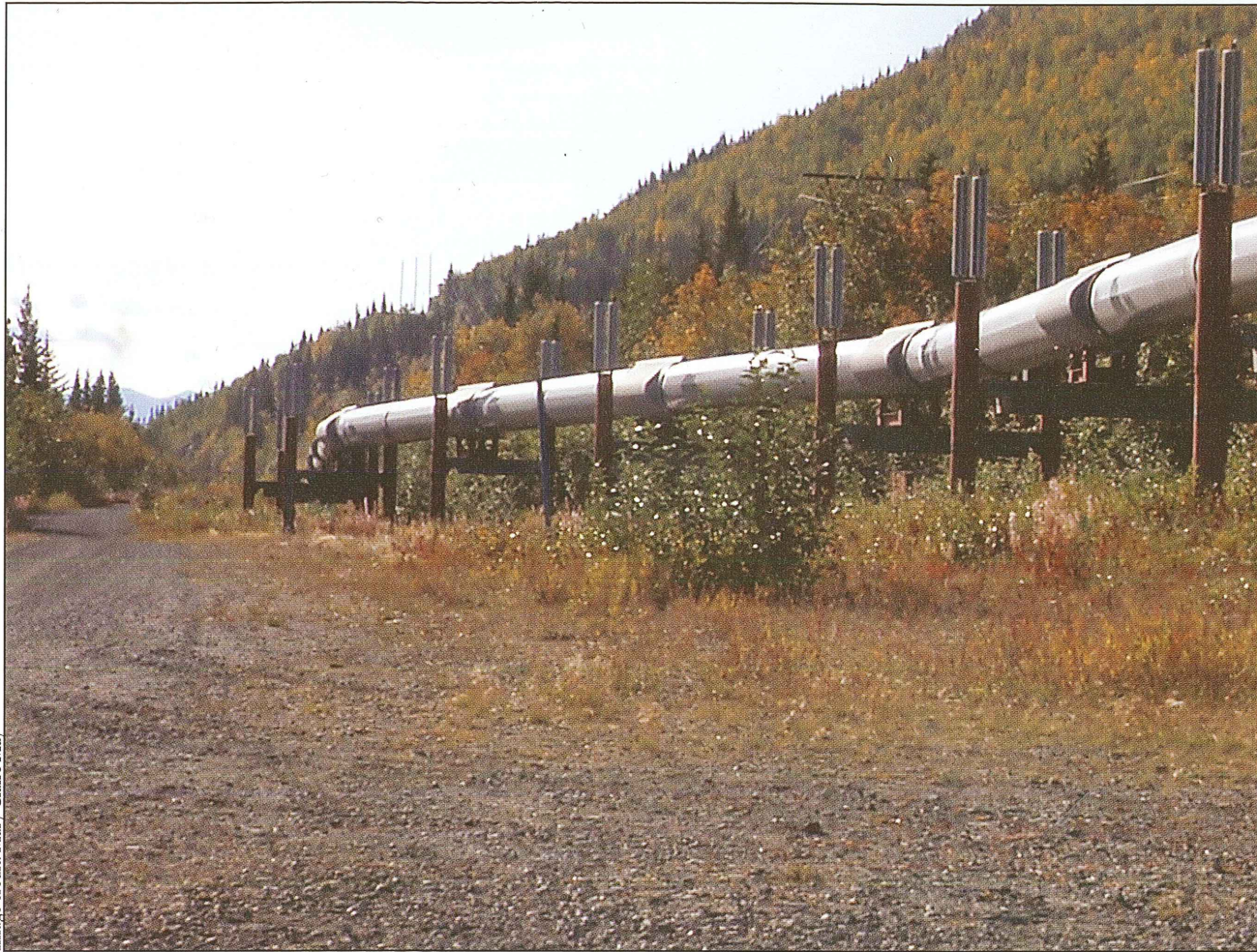
A segment of the 800-mile-long Trans-Alaska Pipeline System winds through the wilderness making connections between Prudhoe Bay and Valdez for the transport of oil.
