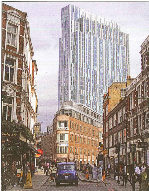
Pointing the way to London’s future, a high-rise dormitory in “The City” contrasts sharply with the low-rise structures characterizing traditional neighborhoods.
