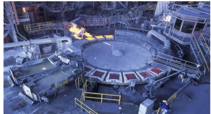
Xstrata Zinc Canada : Bracemac-McLeod Mine Construction
