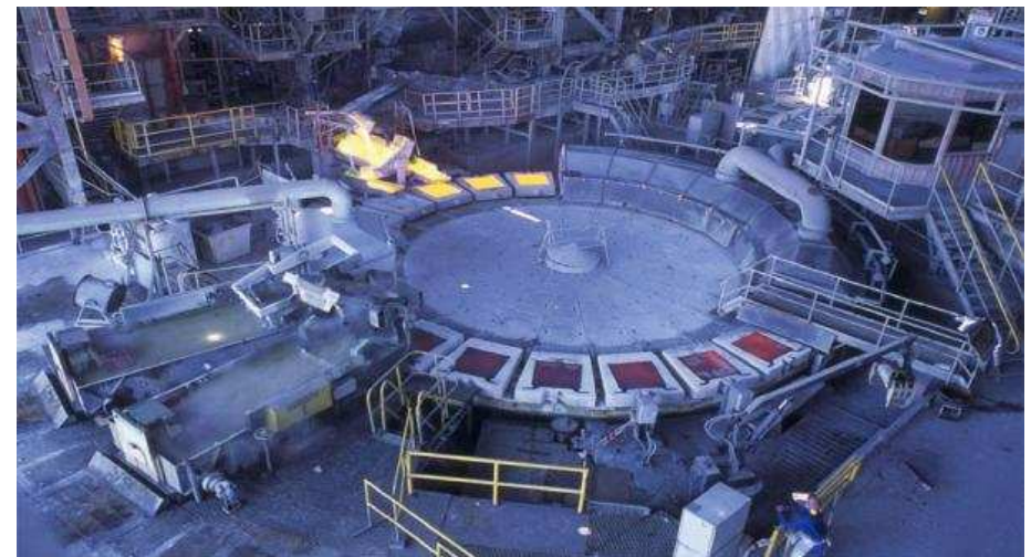
Xstrata Zinc Canada : Bracemac-McLeod Mine Construction
