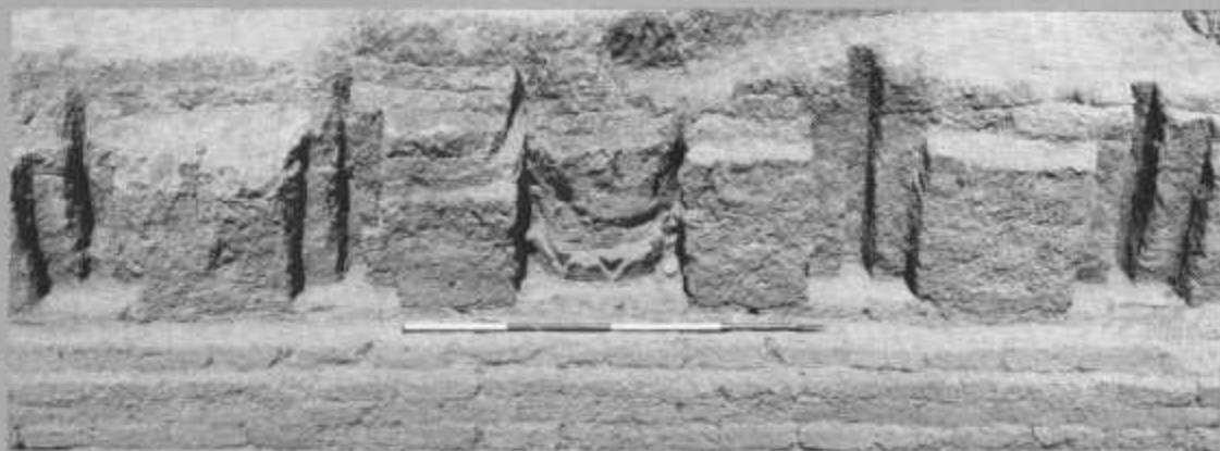
A small portion of the southern facade of the Building Level II temple has thus far been excavated. Like the northern facade it was decorated with niches and engaged columns but was not as well preserved. One mudbrick column was clearly sculpted to resemble the trunk of a "dressed" palm tree.
