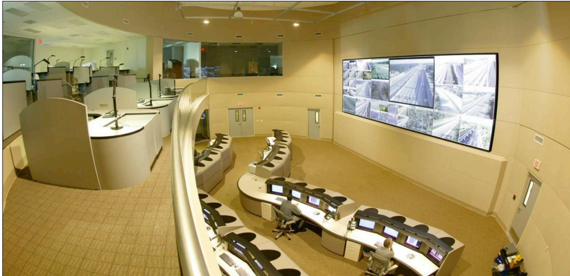
Traffic monitoring, Florida Department of Transportation
