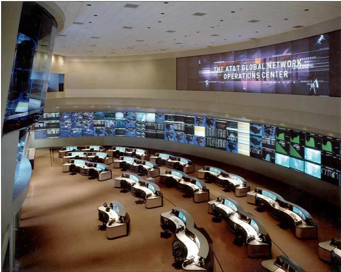
AT&T Global Network Operations Center
