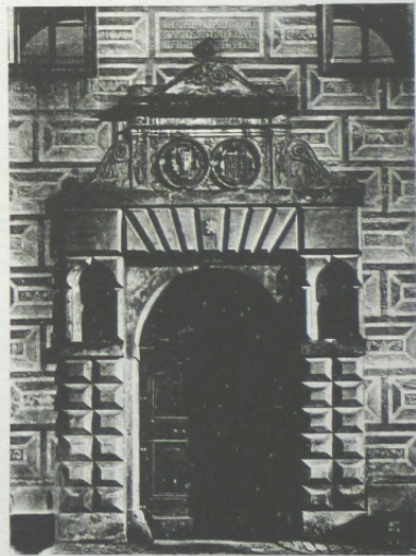
325 Giovanni Battista and Ulrico Aostalli (Avostalis): Main portal and illusionistic rustication, 1568-73, in Litomyšl Castle
