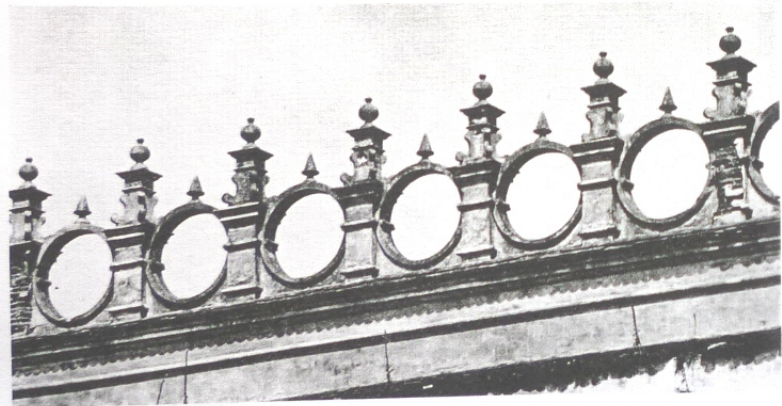
339 Parapet of the south wing of the castle at Krasiczyn (extensively restored early twentieth century)
