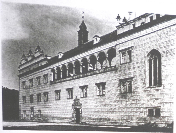
326 Giovanni Battista and Ulrico Aostalli (Avostalis): Loggia of the façade wing, 1568-73, of Litomyšl Castle
