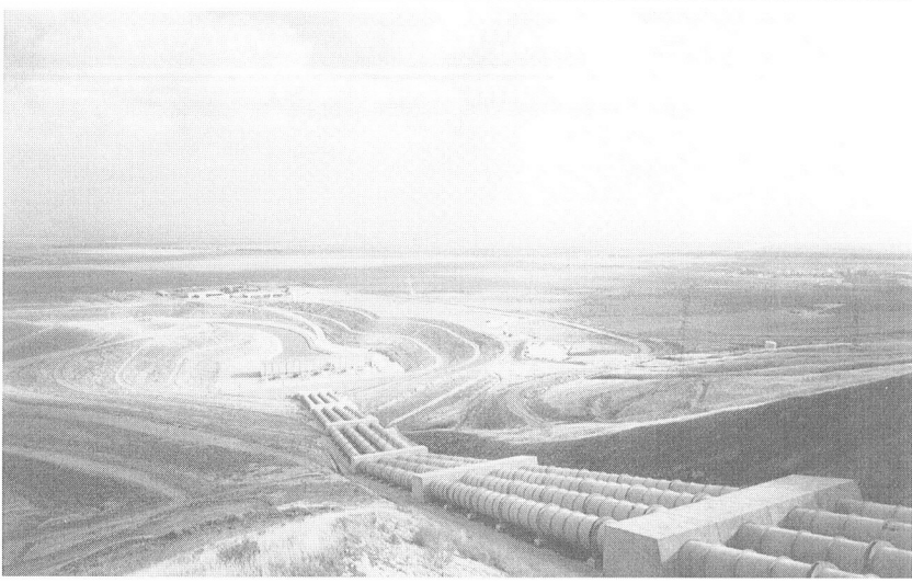
Figure 14: Wind gap pumping station, California Aqueduct, Kern County, 1985. Photo by Stephen Johnson.
