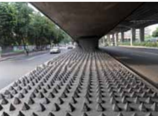
Concrete spikes installed underneath freeway bridges in the city of Guangzhou, apparently intended to deter homeless people from taking up residence.
