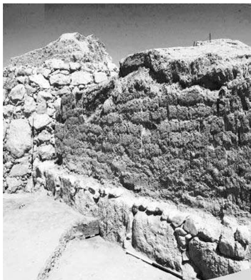
Fig. 4 – Area A: detail of the western foundation wall (W.1659) of MB I-II Tower A1, made of big stone orthostates, and of its foundation trench (P.1687), from south-east.
