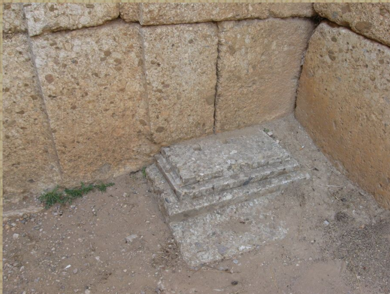
FIG. 21. A method to give the changing slope of the dome of a tholos during construction
