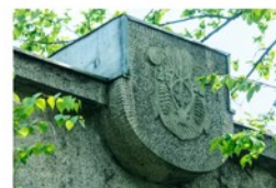
Entrance Building of City Water Reservoir 1 Daleka St
