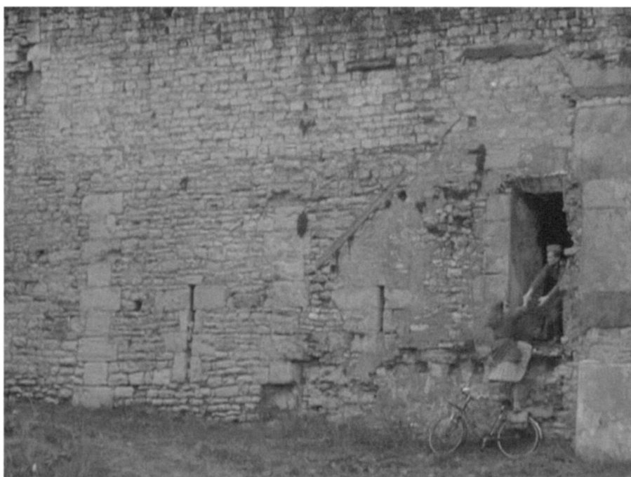
Fig. 10. An entrance in the village wall.
