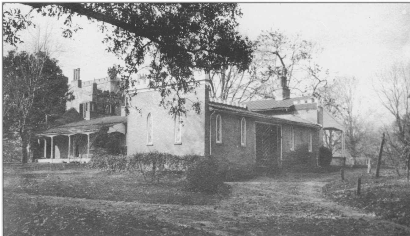
Fig. 14. Staunton Hill, Charlotte County, Virginia. View of service wing, c. 1890. Note the larger, castellated massing of the house beyond. Unlike Berry Hill, Staunton Hill's service wing is linked more directly to the house itself. This link is emphasized visually by the matching Gothic Revival motifs. (Virginia Historical Society, Richmond, VA)
