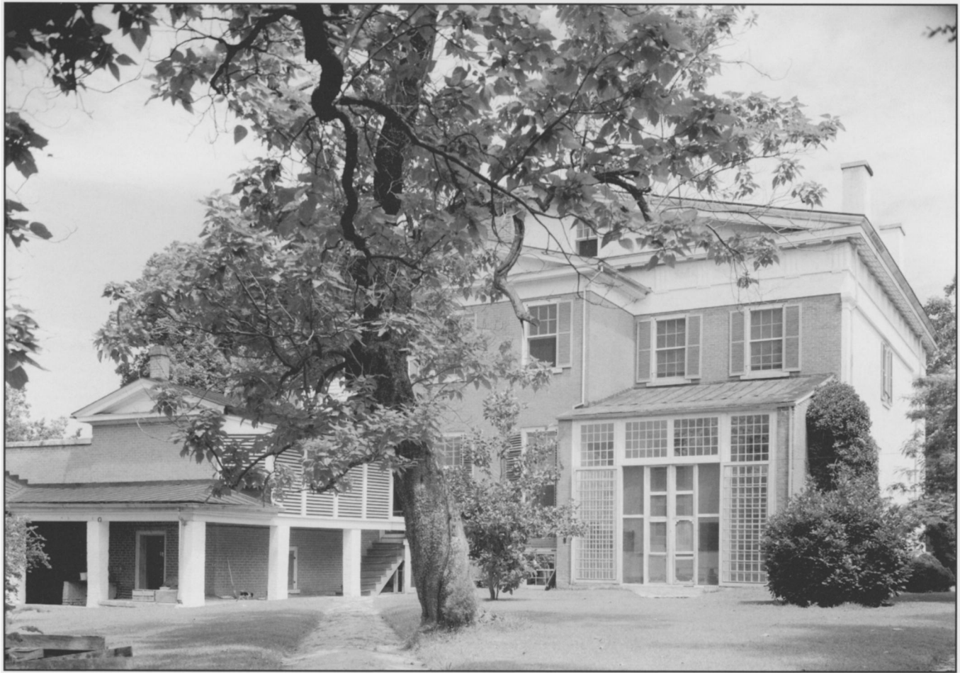
Fig. 9. View of the pantry wing of Berry Hill showing the lowered shed over the colonnade. (Library of Congress, HABS, VA, 42-BOSTS. V, 1-6)
