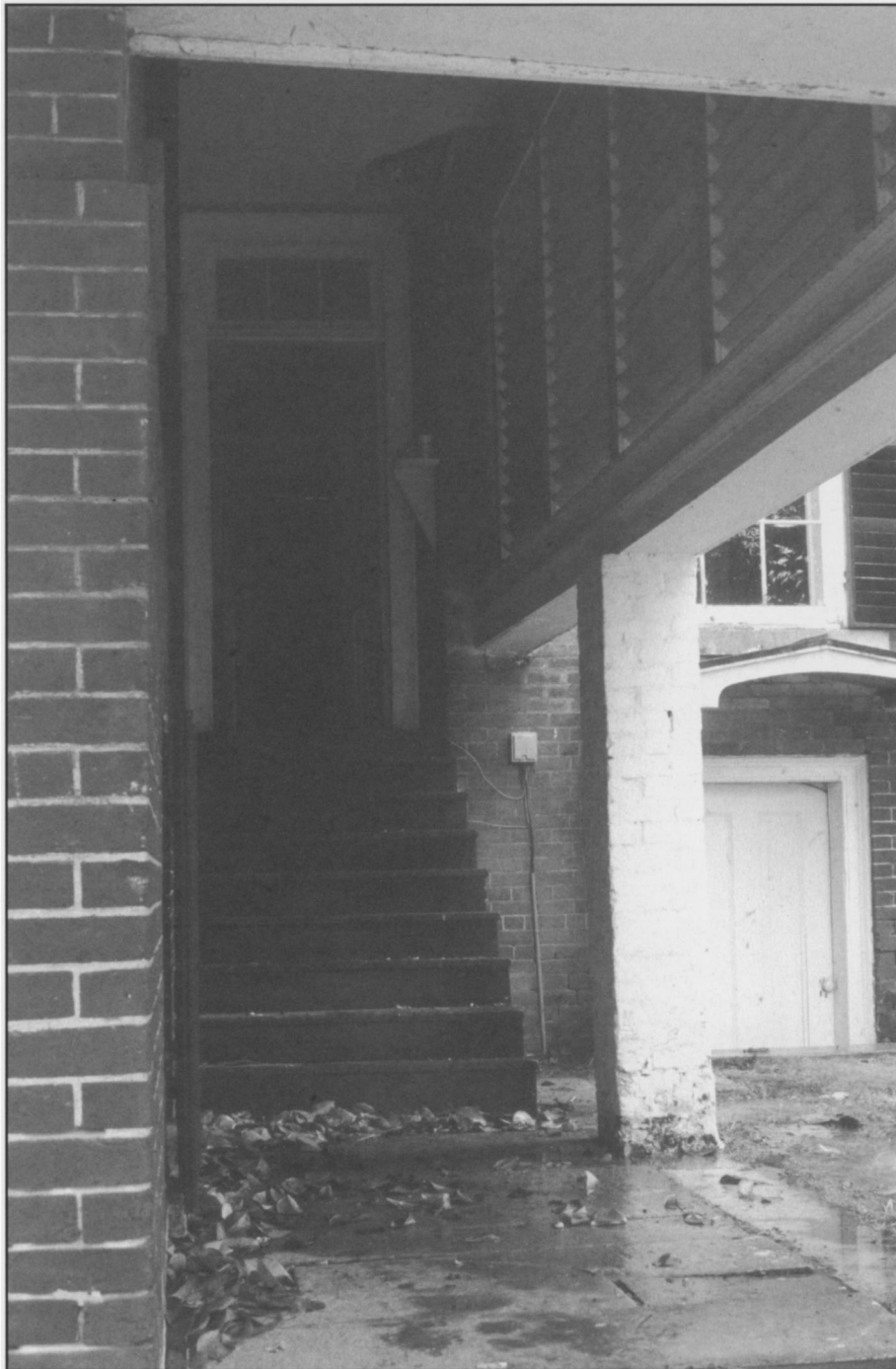
Fig. 10. The lowered shed addition to the pantry wing blocks visual contact between slaves ascending the stairs and the white household otherwise visible beyond the dining room window, partially seen in the upper right. See Fig. 9, exterior view of shed. (Photo: Author, 1999)
