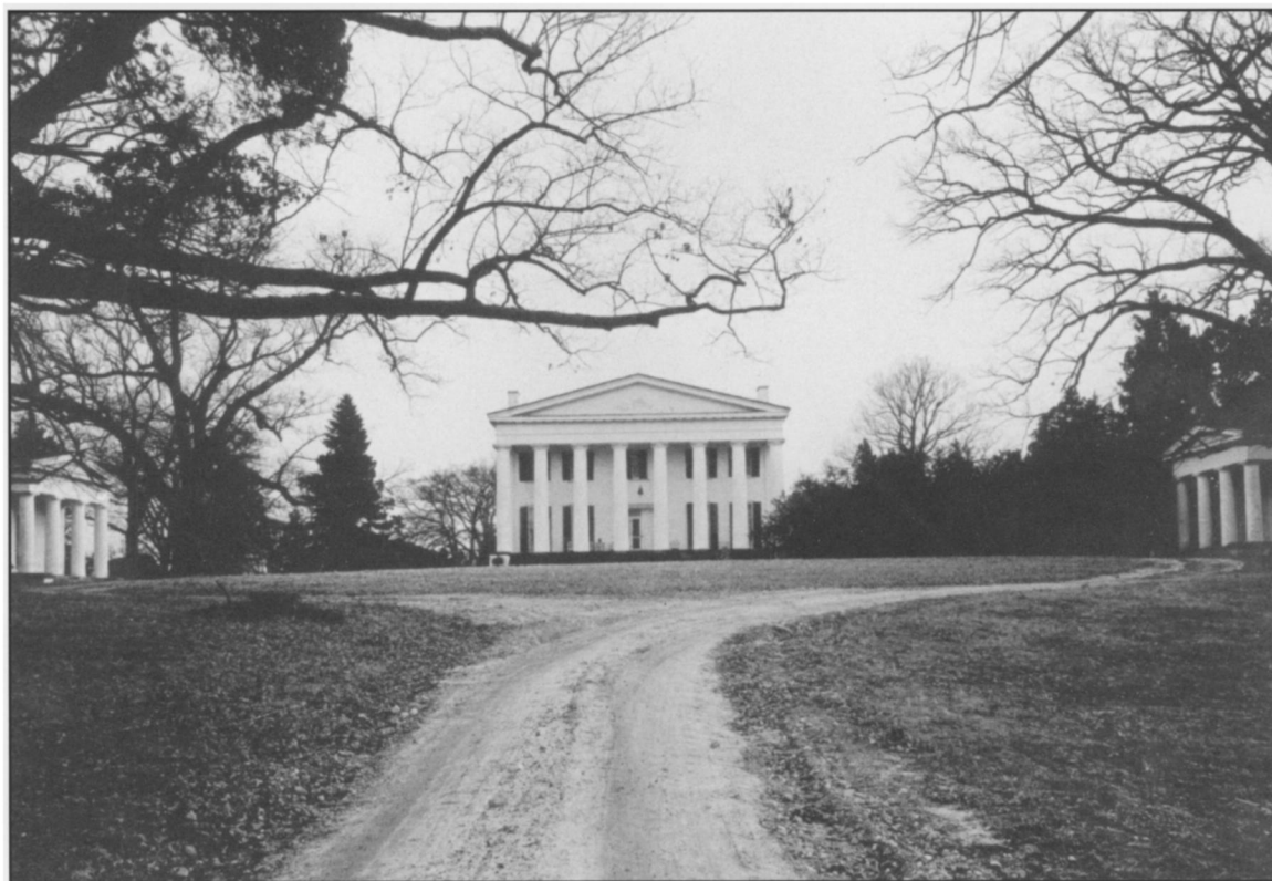
Fig. 1. North elevation of Berry Hill, Halifax County, Virginia. (Virginia Department of Historic Resources, Richmond, VA)
