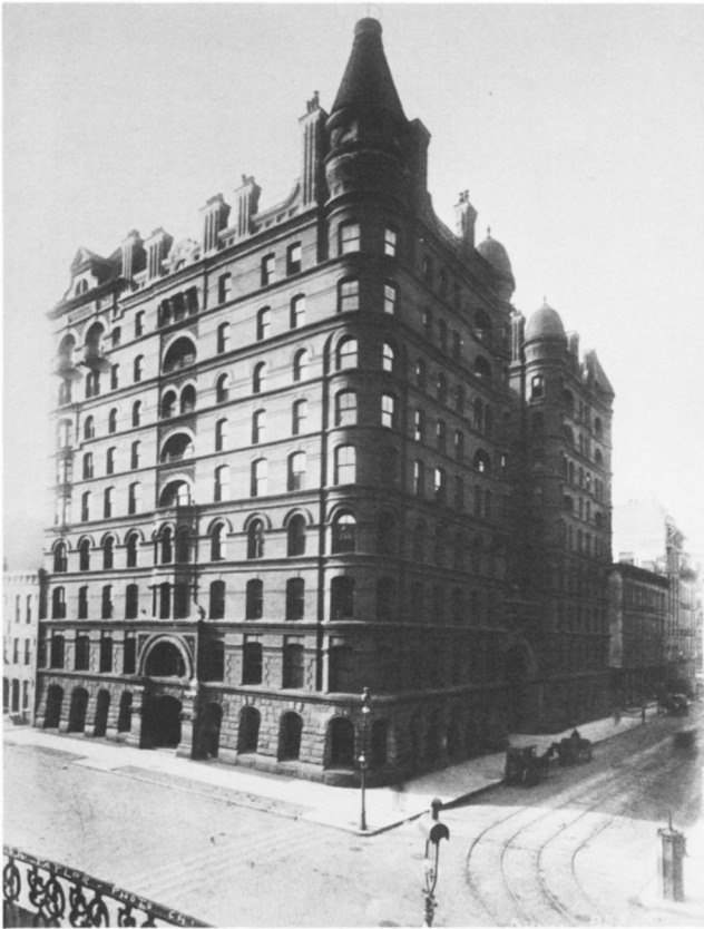
Fig. 2. Solon Spenser Beman, Pullman Palace Car Building, Chicago, 1883. Exterior (J. W. Taylor; Chicago Historical Society).
