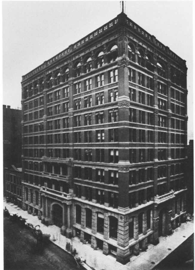
Fig. 1. William Le Baron Jenney, Home Insurance Building, Chicago, 1884. Exterior (J. W. Taylor, IChi-00989; Chicago).
